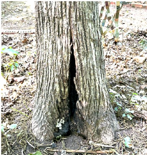
Detail of south side of Subject Tree showing cavity and split in trunk at base of tree.
