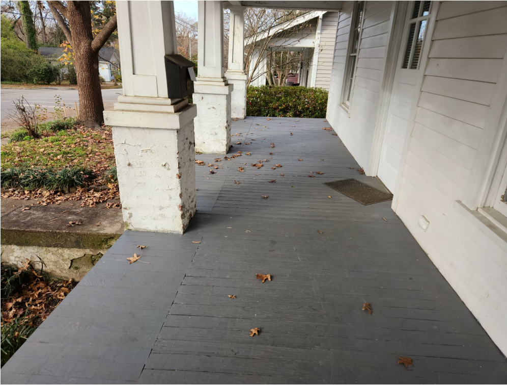
FRONT PORCH FLOOR BOARDS DETERIORATED AND REPAIRED INADEQUATELY
