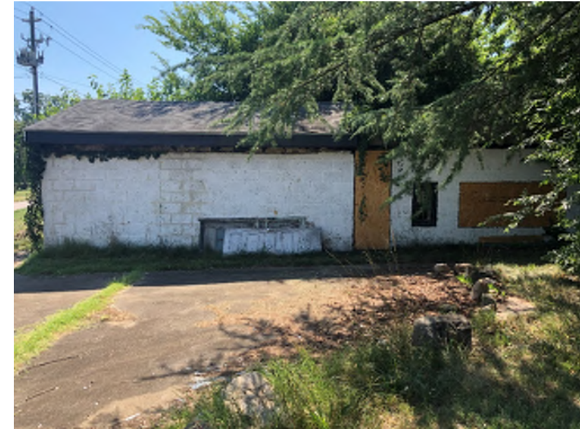
Figure 2: Existing Garage Looking East
