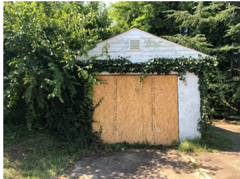
Figure 1: Existing Garage Looking South
