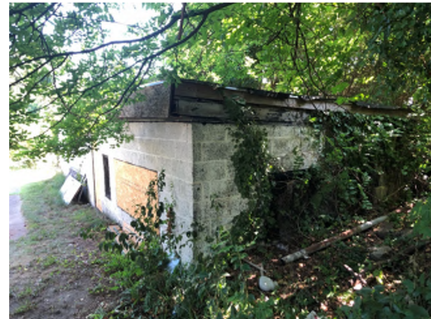
Figure 3: Existing Garage Looking North
