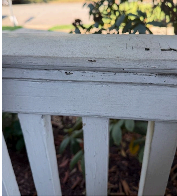
Existing front porch railing — cap and baluster detail.
