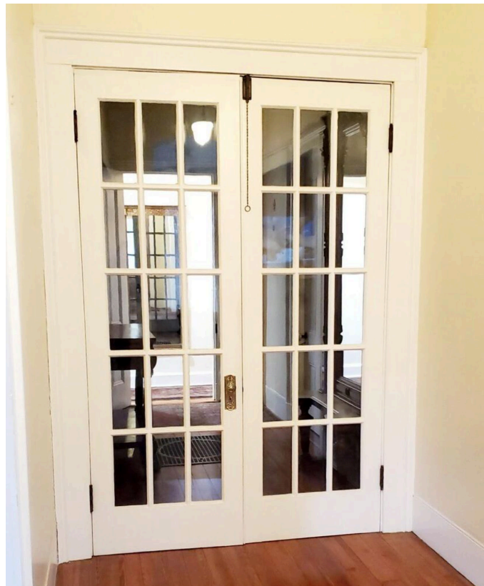
Reclaimed fifteen-light French doors with original mortise lock and brass hardware, salvaged from 318 Oakwood Avenue.
