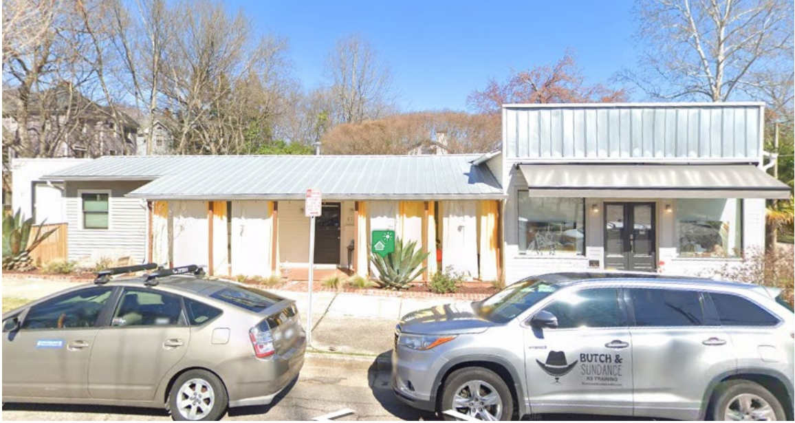
Existing front of home illustrating parapet wall (South view):
