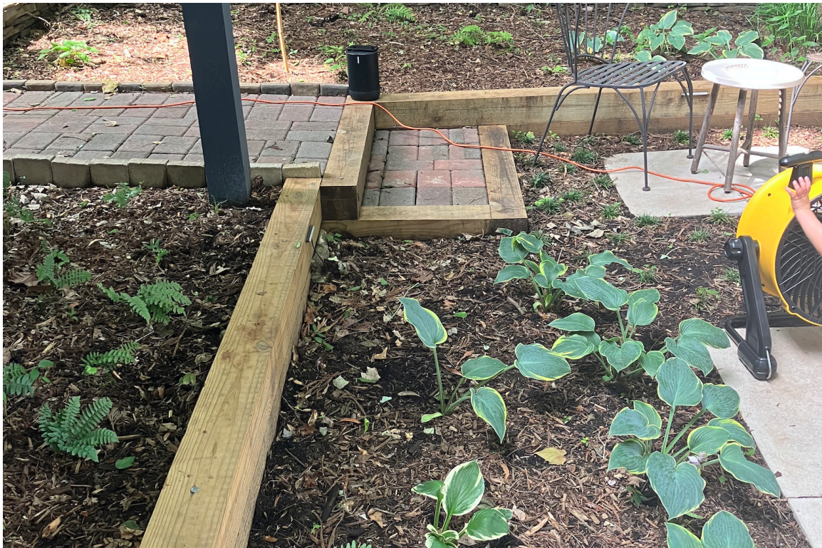
604 N. Bloodworth St. Timber Retaining Wall & Stair
