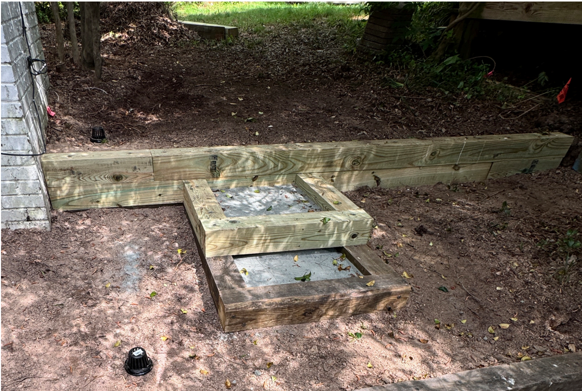
Reference photo of 6"x6" southern pine timber, mixed with exiting timber members
