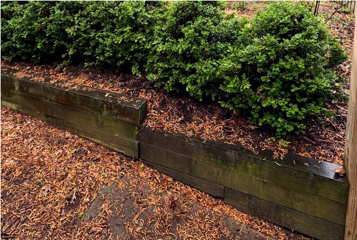
Photo of existing timber retaining wall
