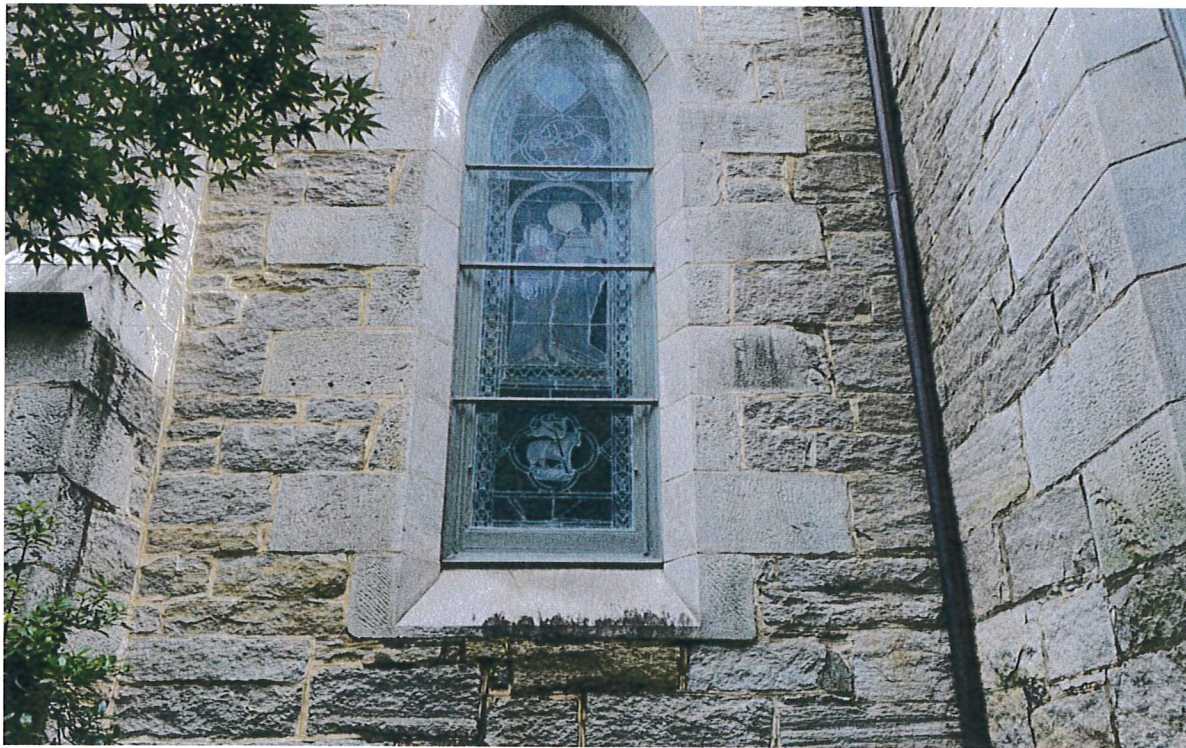
14 – Window Surround Material – Sanctuary south wall
