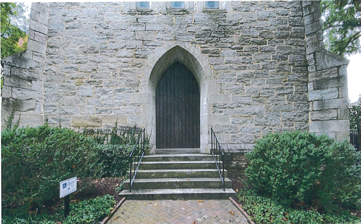
15 – Sanctuary Steps and Arch Surround – From brick walk intersection looking north
