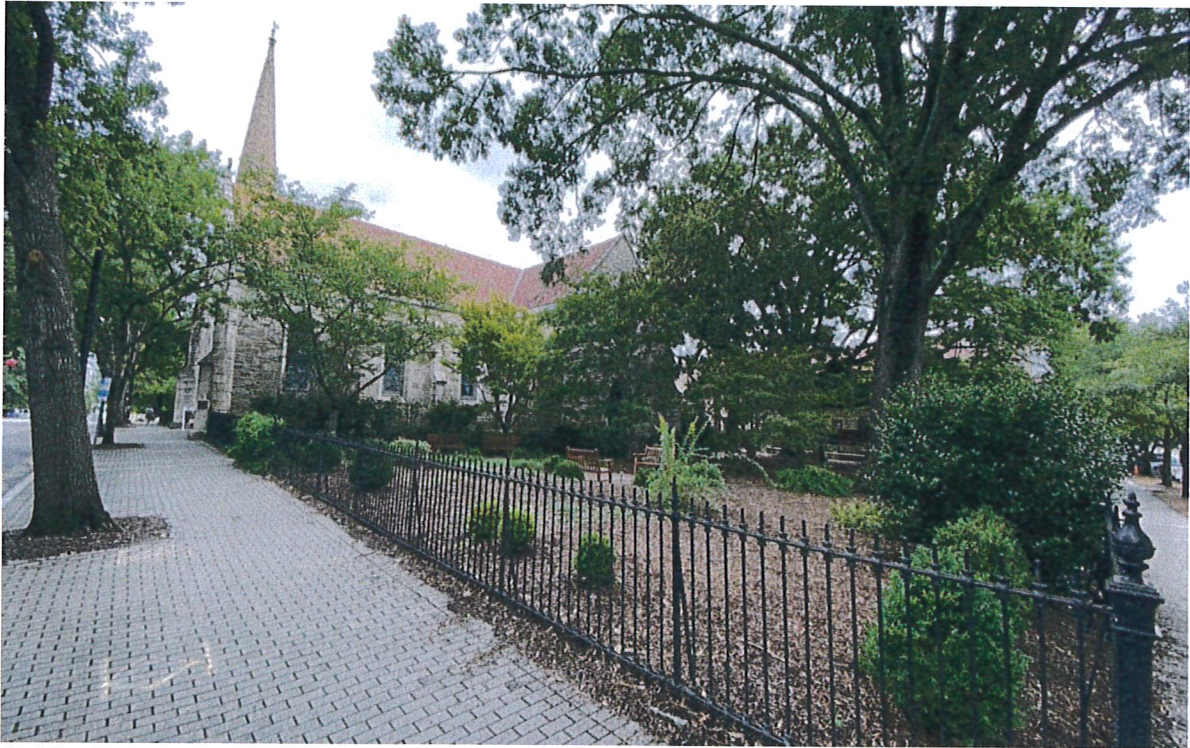
1 – View from corner of N Wilmington St & New Bern Pl – Looking northeast
