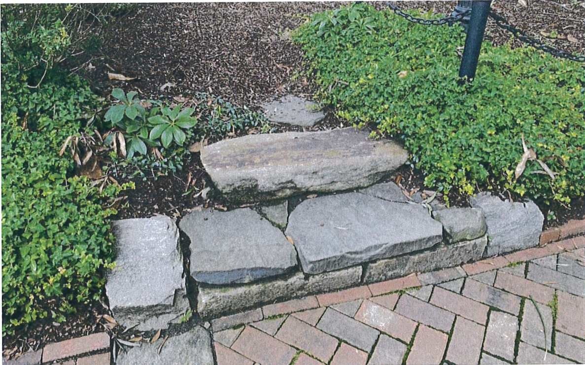
16 – Stone Steps – Near south gate looking west
