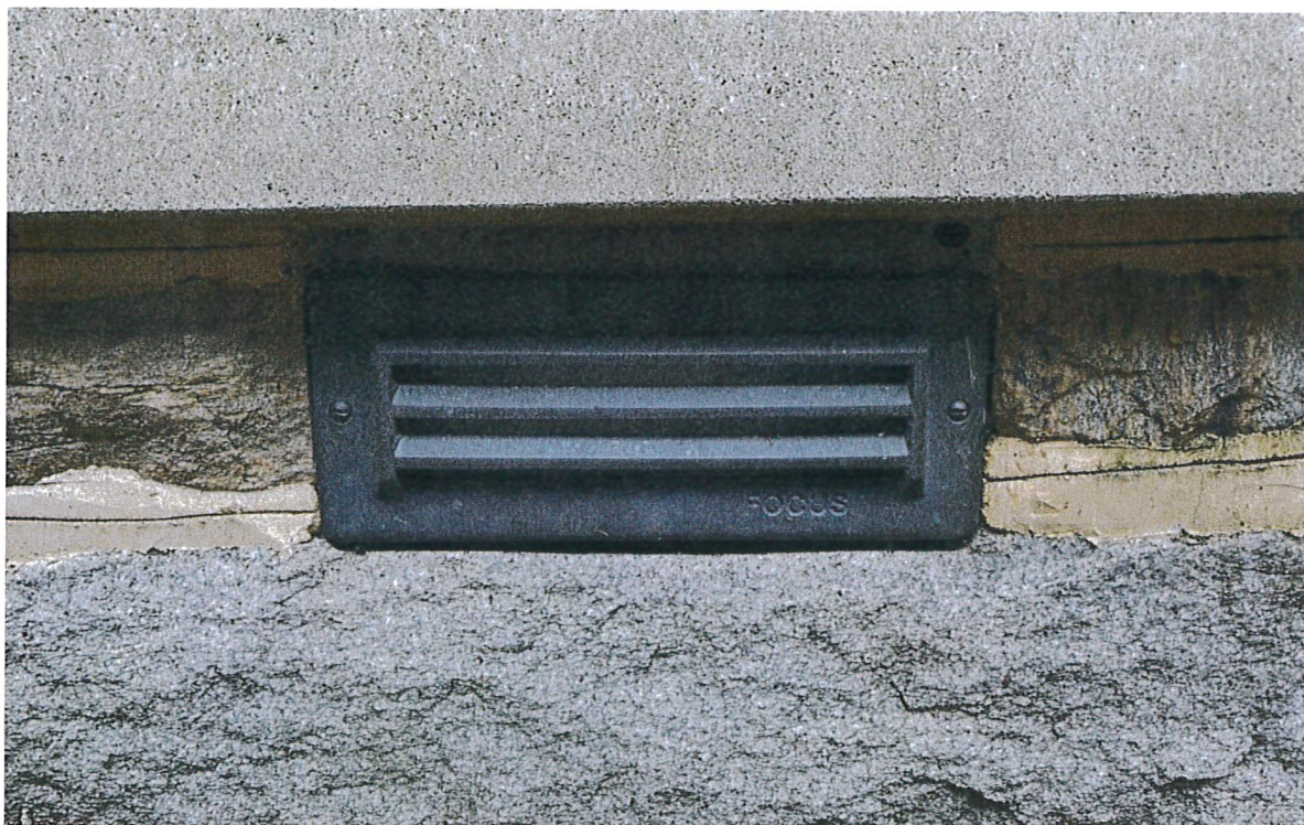
13 – Site Wall at Play Area – Detailed view of existing in-wall lighting
