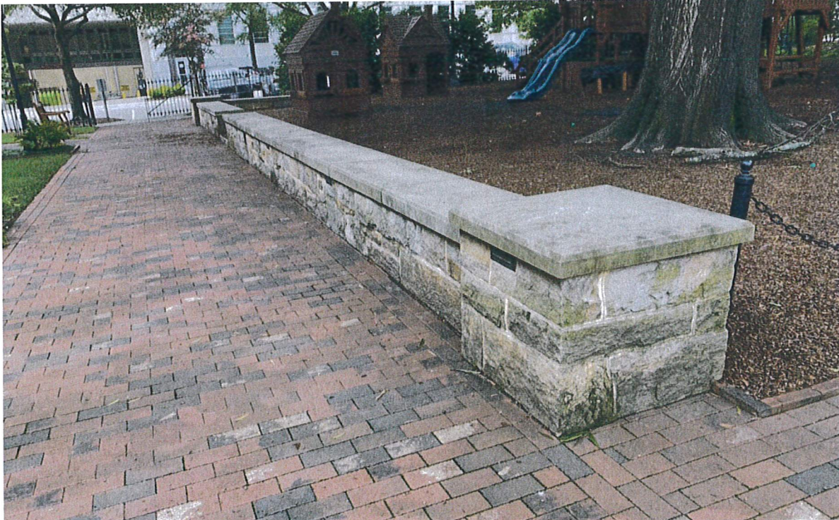
12 – Site Wall at Play Area – From curved path looking south
