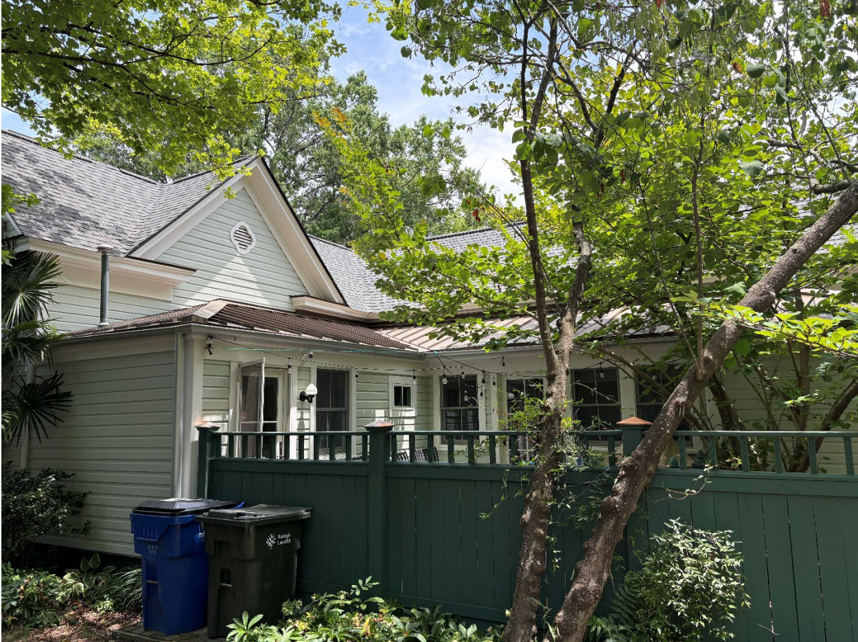
Figure 3. Standing seam metal roof on the back porch of 512 Oakwood Ave. This same brand of roofing is proposed for the front porch at 514 Oakwood Ave. This is 24 gauge standing seam metal roof.
