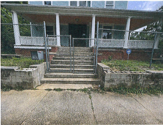
Damages of the existing front concrete stairs and retaining wall capping blocks
