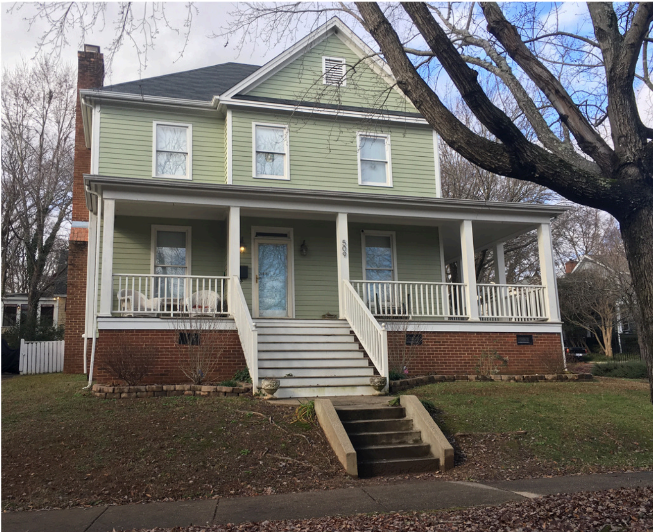
Two and a half story house with a hip roof and front dormer
