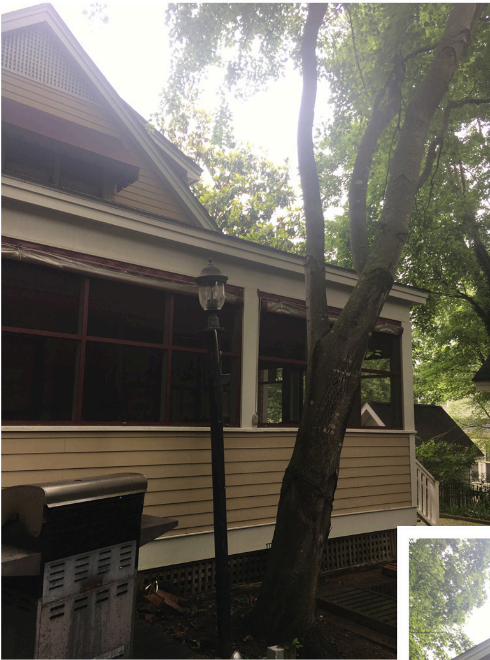
Rear of house and tree that we will remove
