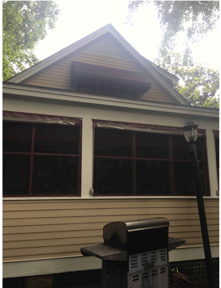
Rear elevation of house
