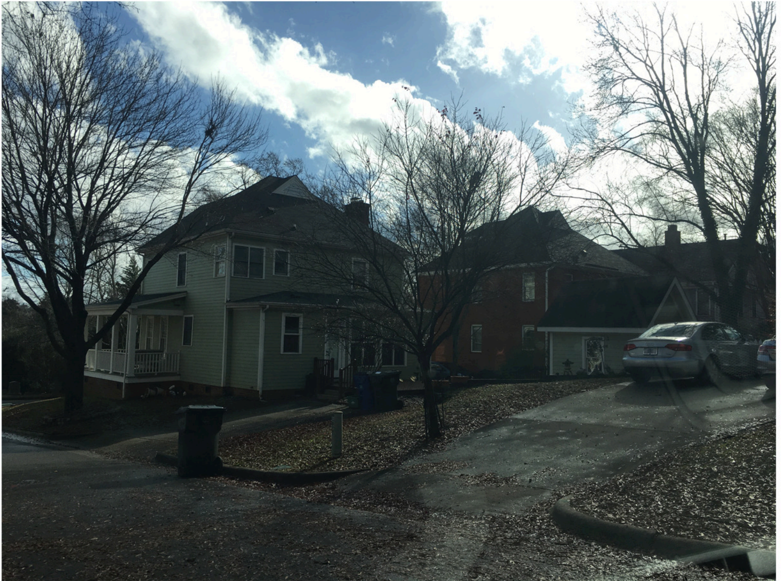
View of 509 + 505 Watauga from Latham Way driveway 600
