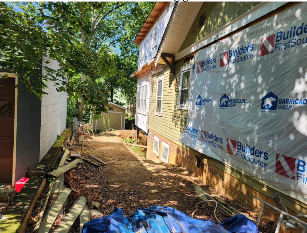
10-Northeast view of Elevation
