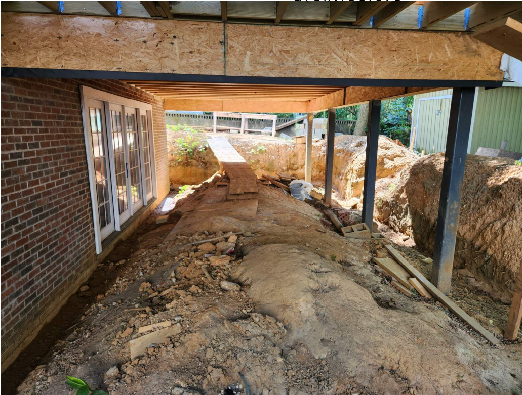
5-West view of Covered Patio before final grading
