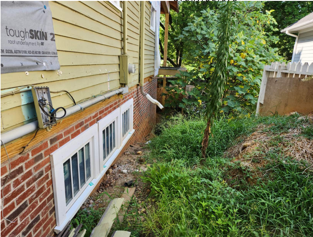
3-View North along West Façade showing grade.
