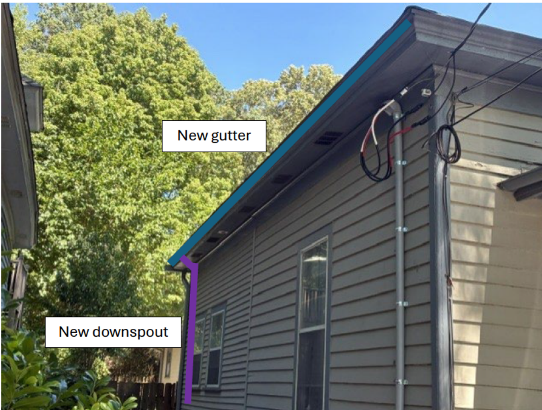
Left (north) side of house
