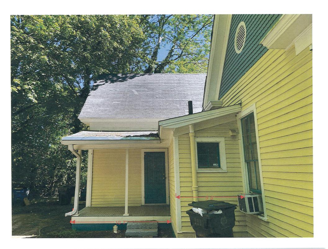
New rear double door to be custom made by vintagedoors.com, recommended by Period Homes online. To be ordered slab only so that sills/jambs can match existing entry door. Transom window to be framed out as single 16" window with glass pane. Trim will be painted white to match the rest of exterior.
