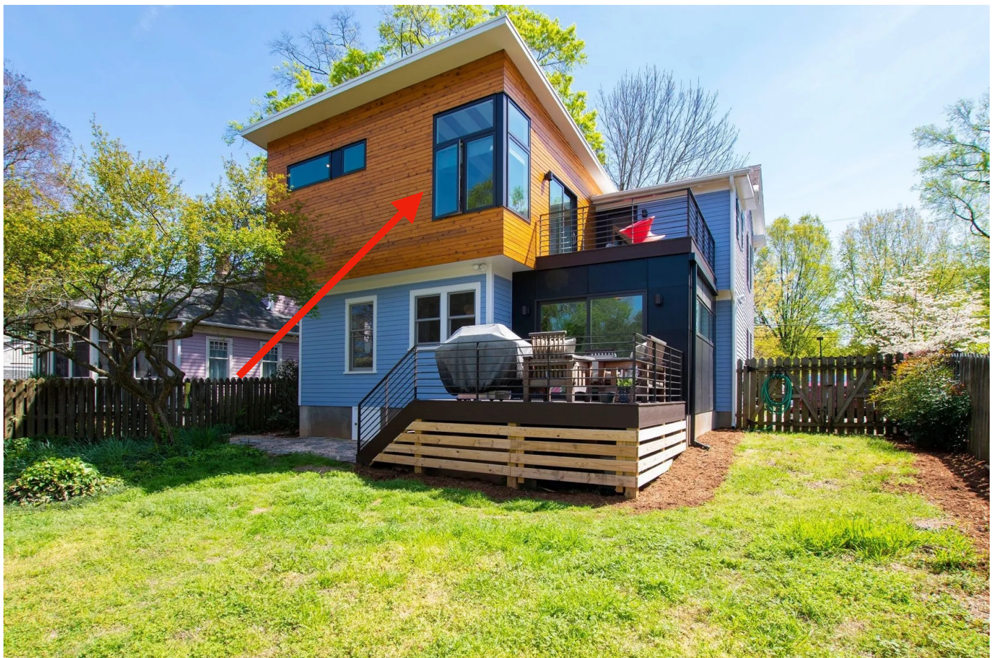
622 Devereux St - window design and siding material on historic addition
