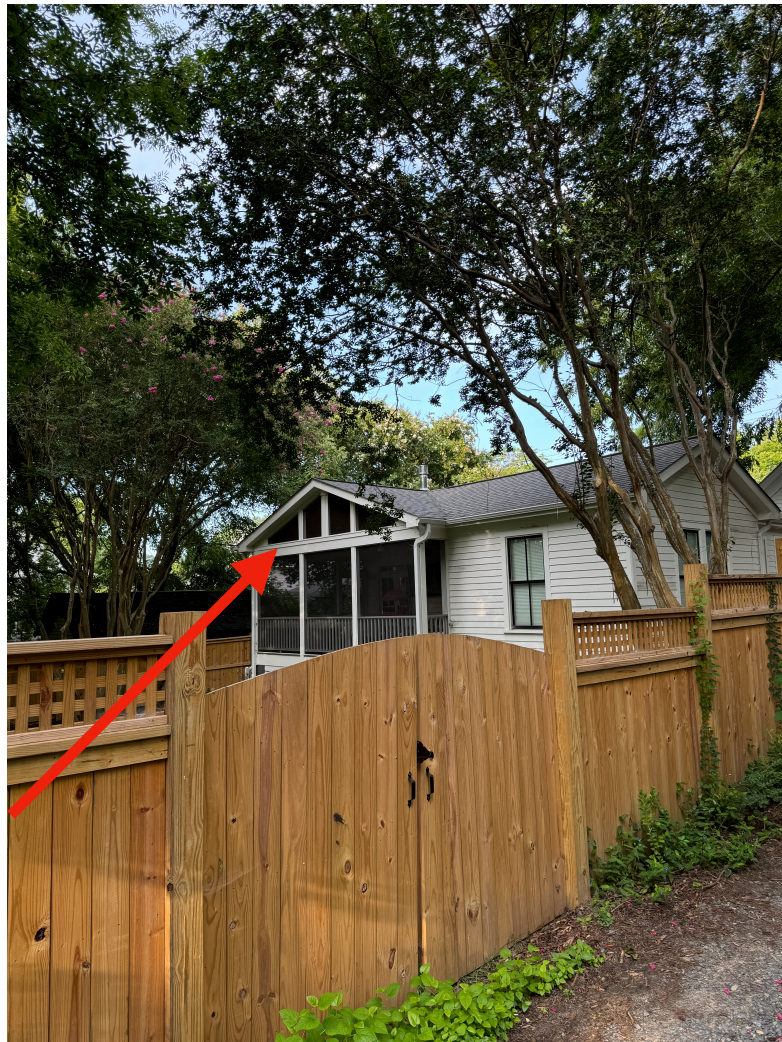
410 N East St - screen porch addition with triangle design element
