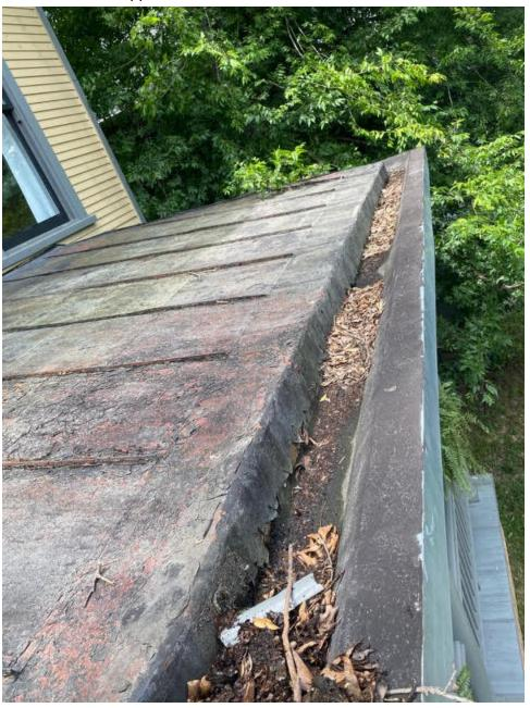
Picture shows a double standing seam hip (nice detail rarely seen nowadays); Siding to be removed to tuck copper flashing appropriately, replace siding with new, will show more pictures where shows signs of deteriorated siding not worth keeping.
