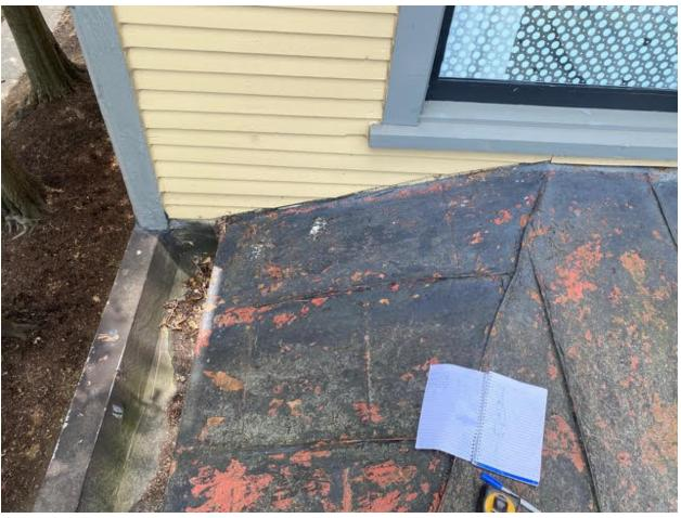
Siding splitting, once we try to pry out wood, prone to break. For watertightness suggest to have replaced with new siding.
