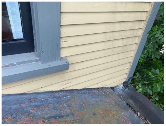
Heavy sediment formed at the bottom of built in gutter.
