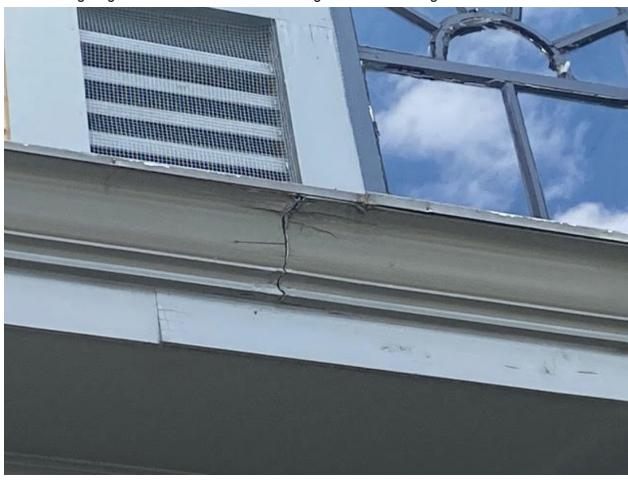
Both downspouts will leave in place, can make new drains from the top and properly solder to insure watertightness.
