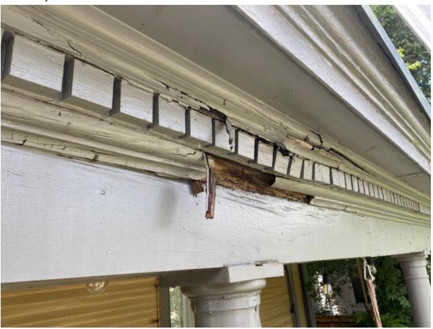
Roof and built-in gutter shows some repairs were made but accumulation of dead leaves and sediment might have been a problem that accelerated the corrosion process. What you have was a nice roof, most likely original with proper folding techniques but with tin/tern coated steel (material failure), is time to replace with a long lasting material that will not corrode, suggested material: 16 OZ copper.
