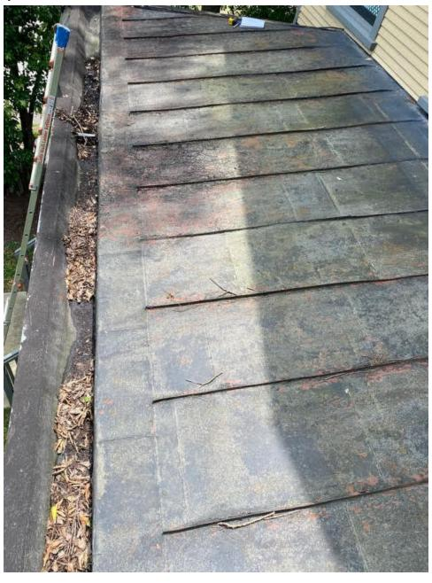
Found a couple of holes, set my ruler to give an idea of size, these located around the center and to the right of porch roof. Soffit underneath shows cracks on wood.
