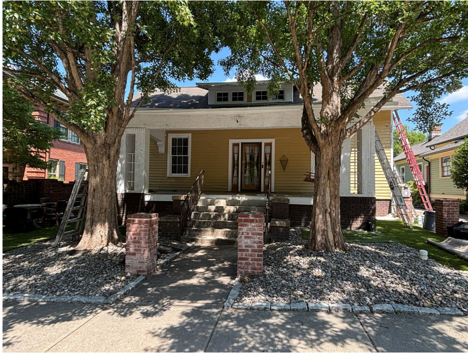
Existing Conditions - 728 N Blount Street; 2026-07-01
