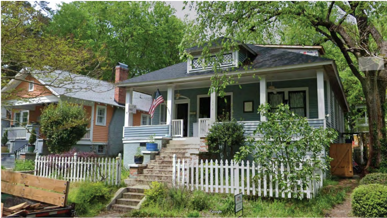
904 SOUTH ST : HIP ROOF STRUCTURE WITH HISTORICAL FRONT DORMER, AND NEW SIDE DORMERS
