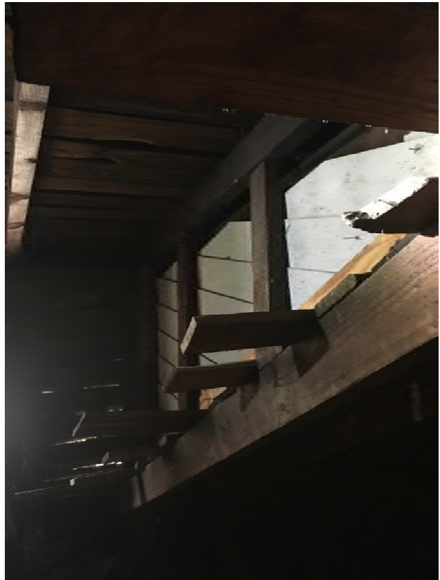
518 SOUTH BOYLAN AVE : FRONT DORMER SHOWING GAPS & DECAY OF EXTERIOR SIDING, AND NO SHEATHING; SIDEWALLS BUILT ON ROOF STRUCTURE WITH NO SUPPORT BELOW.
