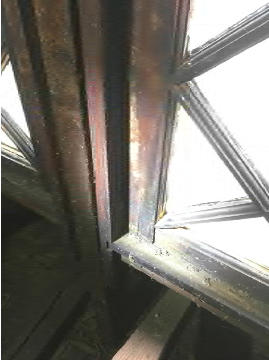
518 SOUTH BOYLAN AVE : FRONT DORMER WINDOWS WITH GAPS AND DECAY TO BE REPAIRED
