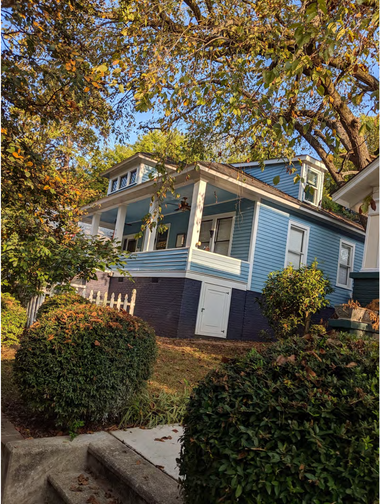
904 SOUTH ST : HIP ROOF STRUCTURE WITH HISTORICAL FRONT DORMER, AND NEW SIDE DORMERS
