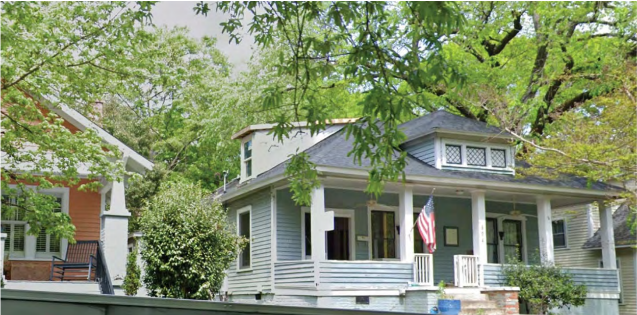
904 SOUTH ST : HIP ROOF STRUCTURE WITH HISTORICAL FRONT DORMER, AND NEW SIDE DORMERS
