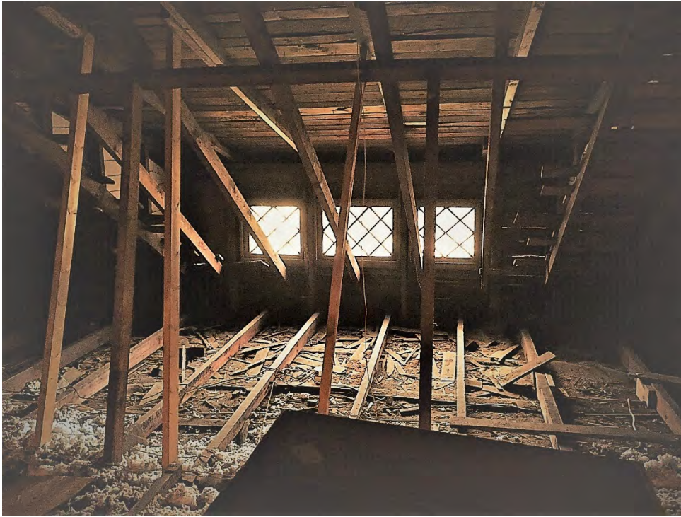
518 SOUTH BOYLAN AVE : FRONT DORMER SHOWING EXTRA POSTING TO STRUCTURE
