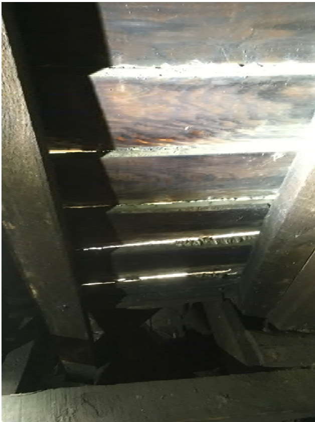
518 SOUTH BOYLAN AVE : FRONT DORMER SHOWING GAPS & DECAY OF EXTERIOR SIDING, AND NO SHEATHING; SIDEWALLS BUILT ON ROOF STRUCTURE WITH NO SUPPORT BELOW.
