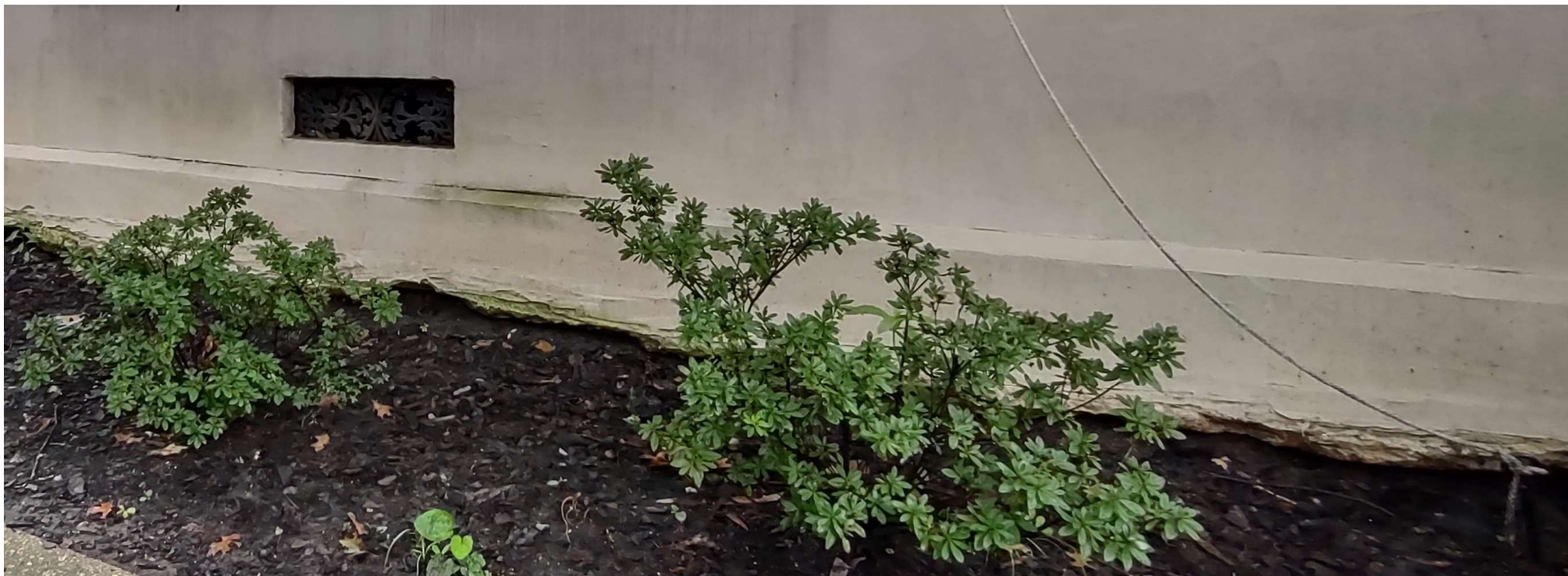
Deteriorated stucco along the base to be patched; this occurs around the entire base of the structure.
