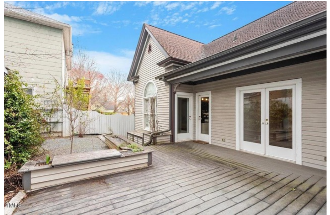
Current Pictures Of The Roof
