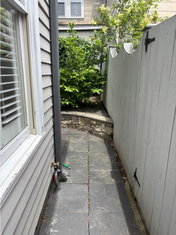
East side of property looking North to backyard
