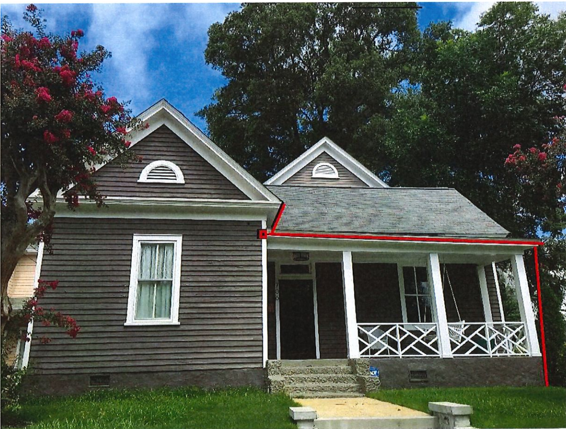
Front gutter placement
