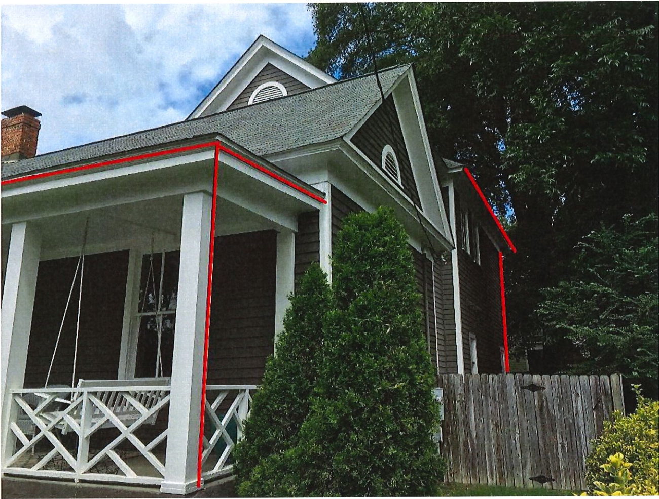
Right side gutter placement
