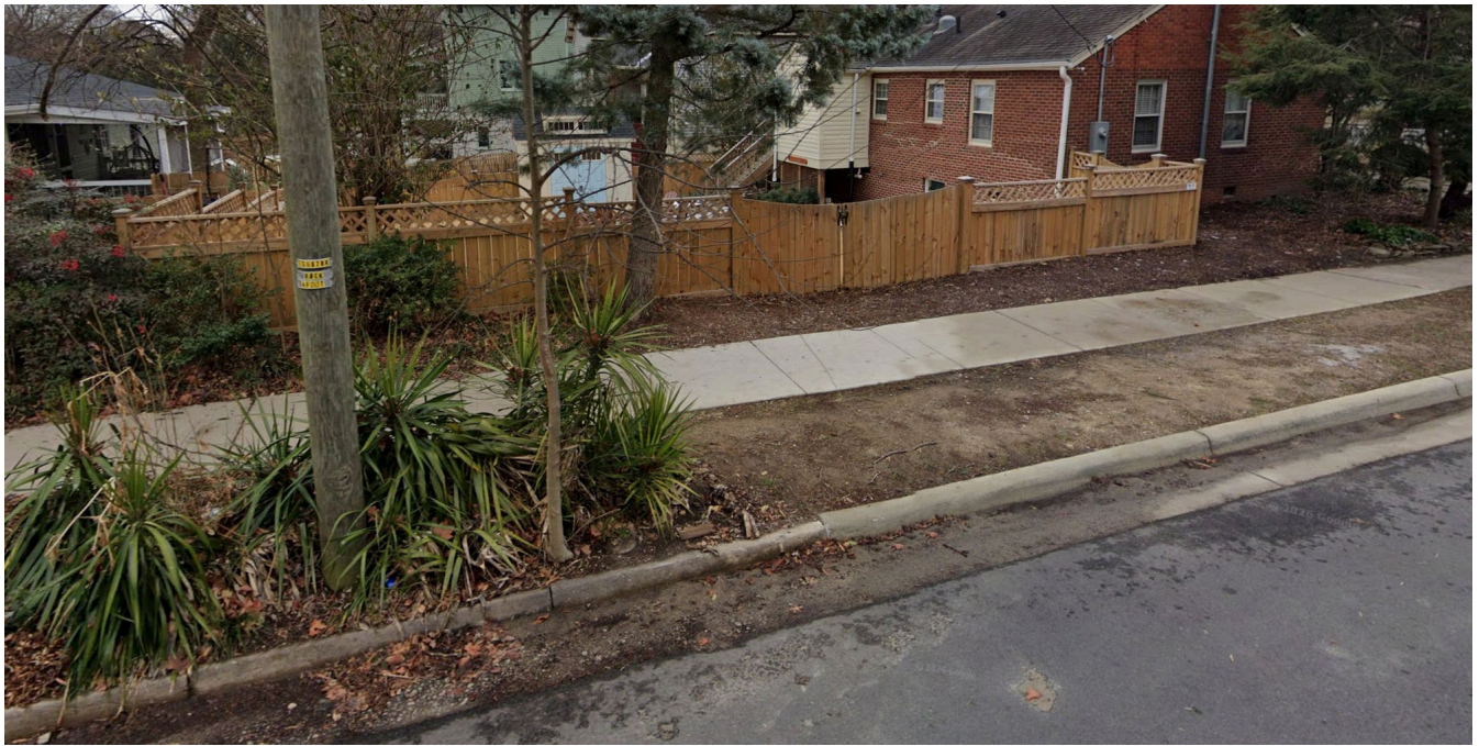
501 N. Boundary Street — completed fence, street view (approved under COA 062-15-CA)
