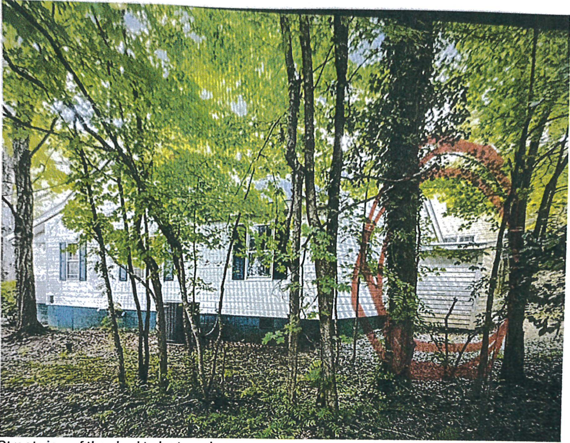
Street view of the shed to be torn down.
