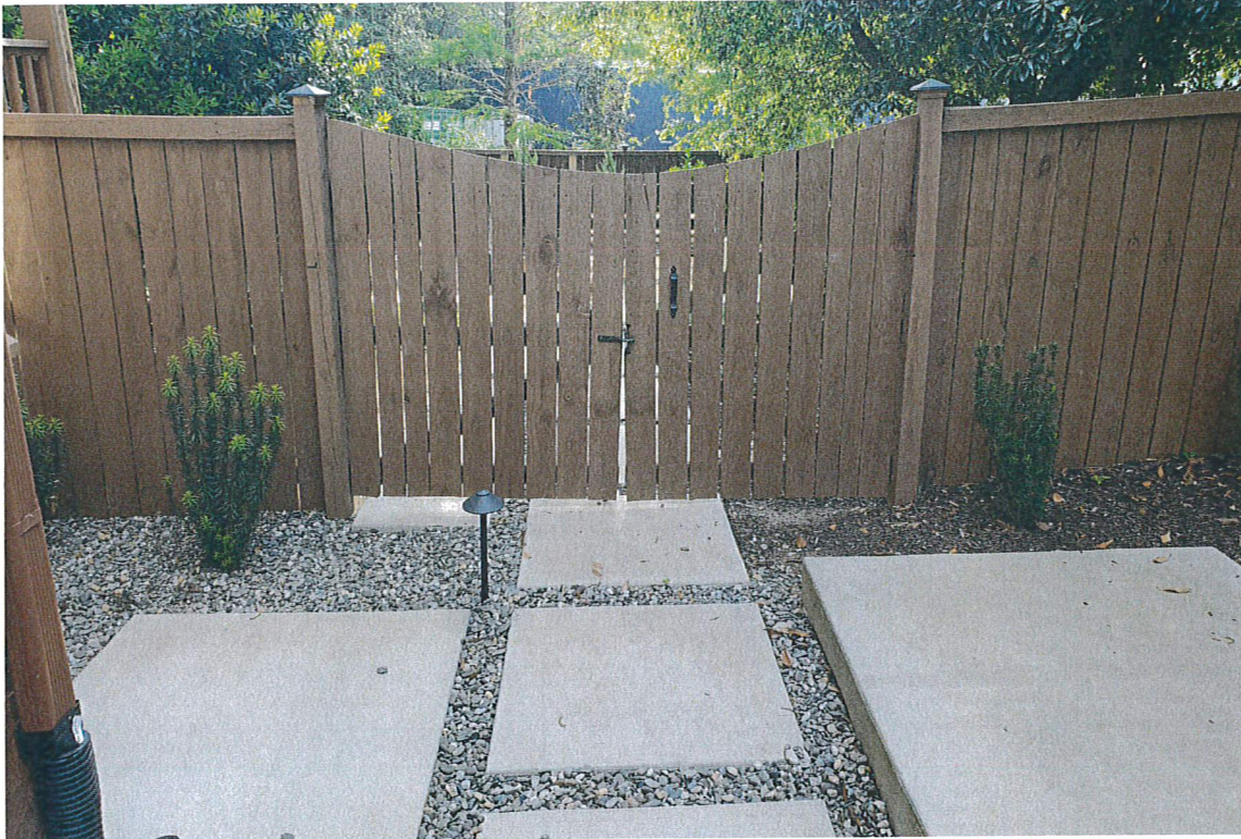
Photos of Existing Broom Finish Concrete Pavers
