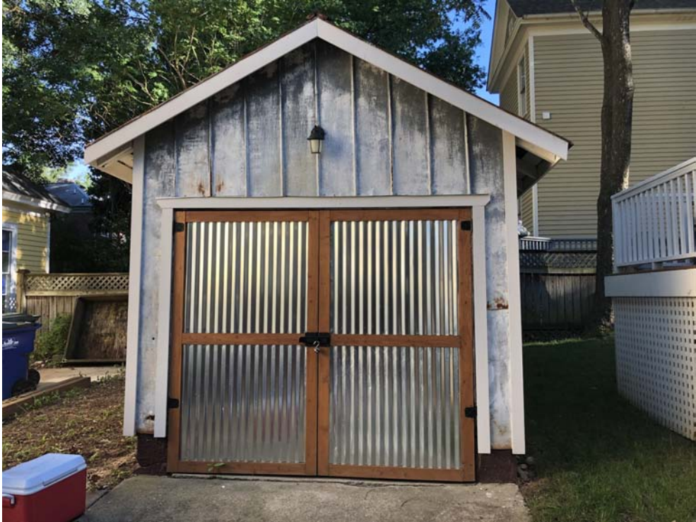
Existing metal shed to be demolished - Street side facing E Jones St
