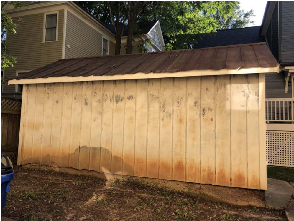
Existing shed - East Side facing concrete pavement and neighbor
