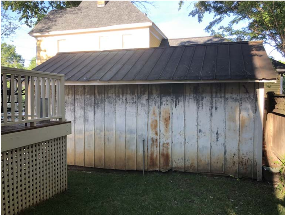
Existing shed - west face against deck and house
