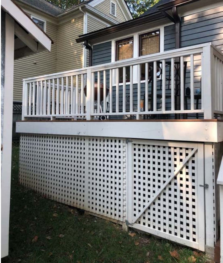
East side of house - Existing Deck
