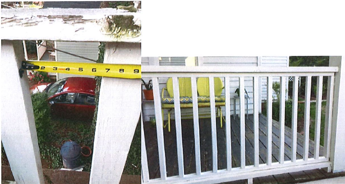
(left) upper railing baluster spacing; (right) lower railing
