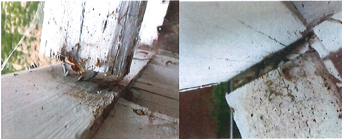
The two attachment points of the current railing. 2 nails per, and not entirely embedded.
