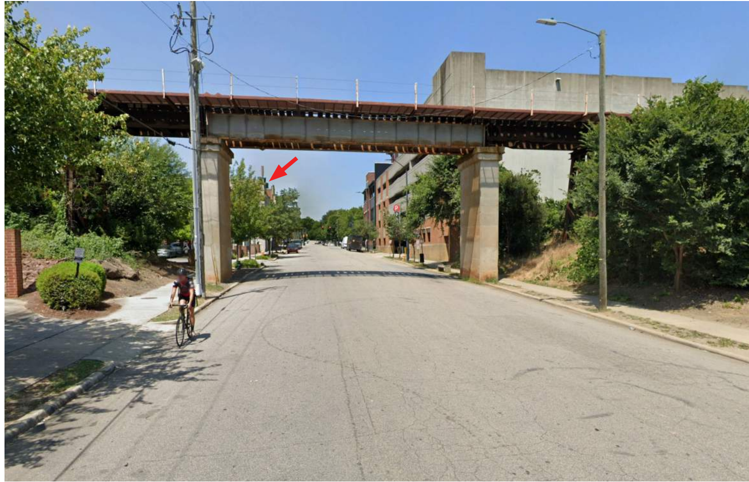
G View looking west down Tucker Street. The railroad bridge and embankment in the foreground obscures views of the Pine State Creamery building beyond.
