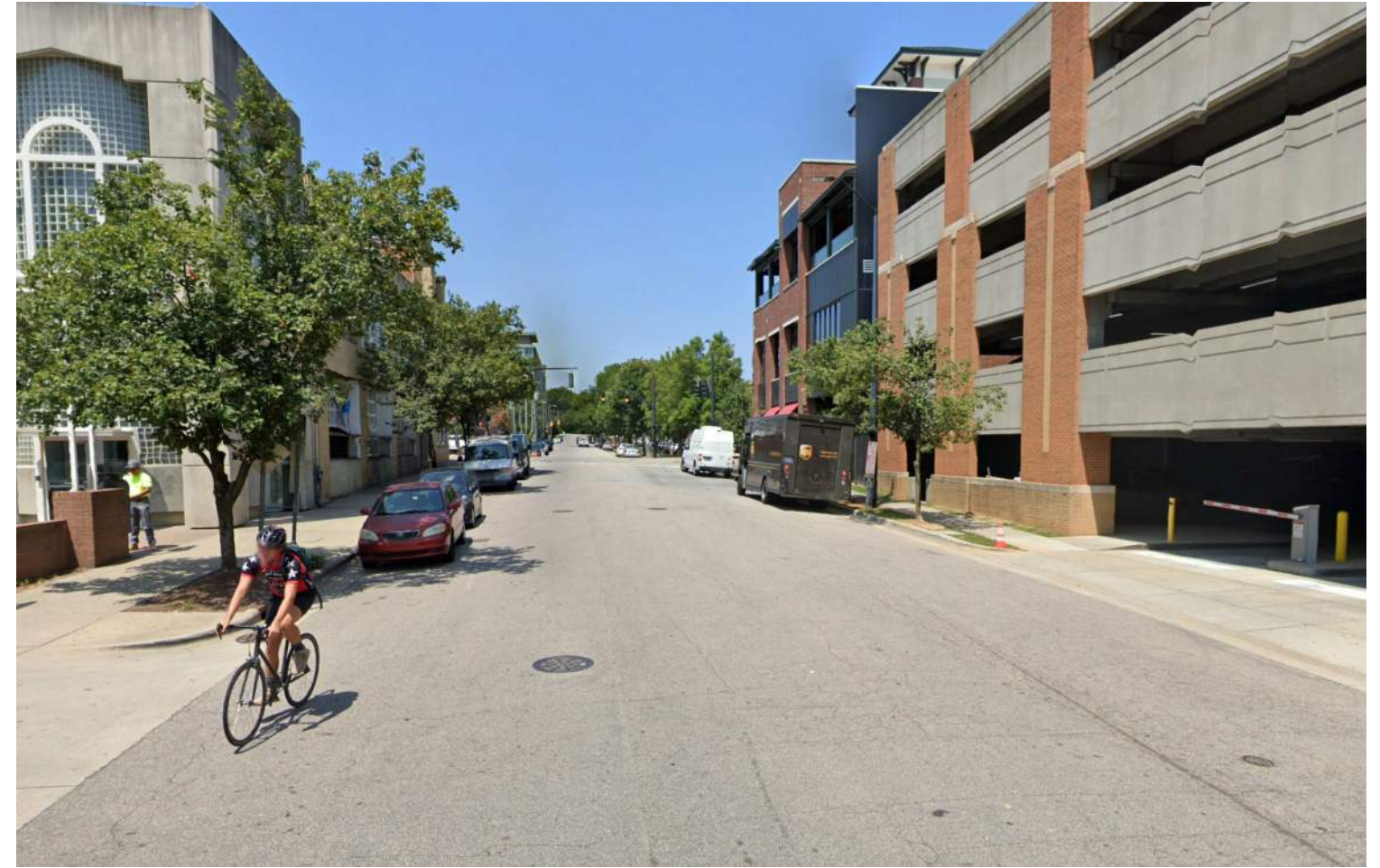
H View of the surface parking lot adjacent to the Pine State Creamery looking west on Tucker Street (East Elevation). The historic 1928 portion is obscured by the 1998 addition.
