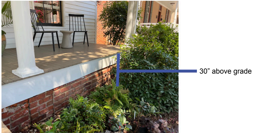
Image 3: Current View of Porch Height
