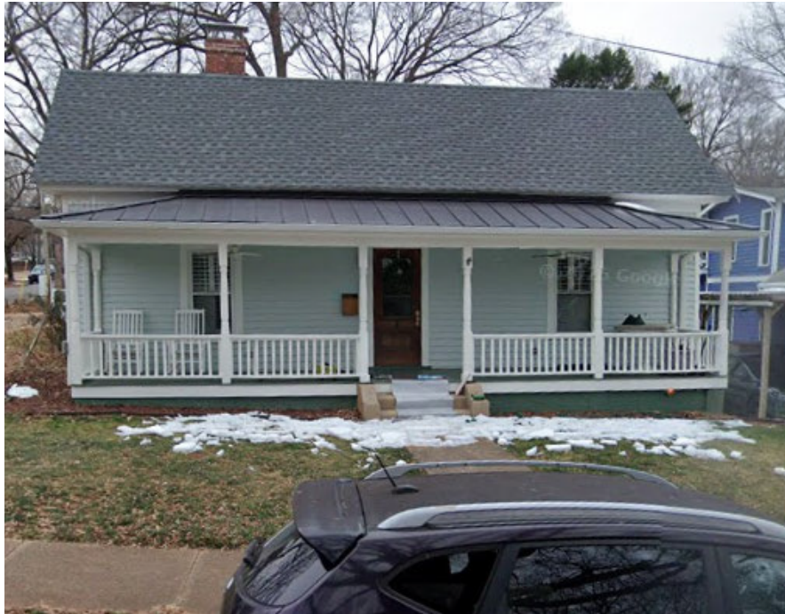
Image 11: 1301 Filmore St. (Architecturally Comparable Home on a Nearby Block)
