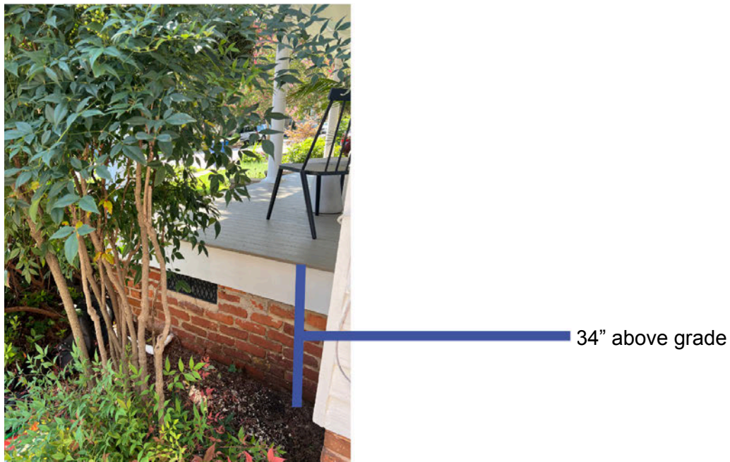
Image 2: Current View of Porch Height
