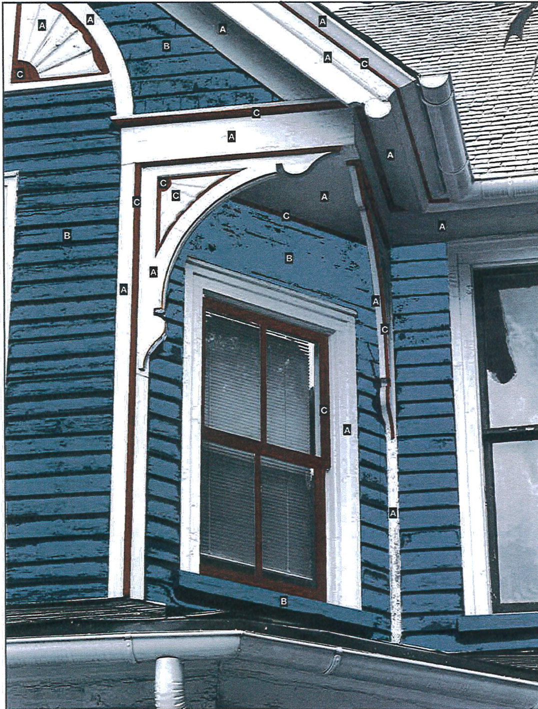
Second floor window and clipped corner color locations.
