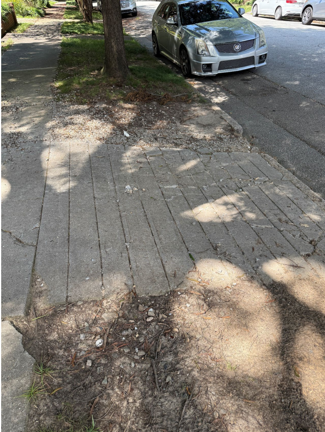
Existing Broken Concrete Apron
