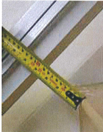
RAIL TO STEP NOSE MINIMUM OF 3 1/4"
