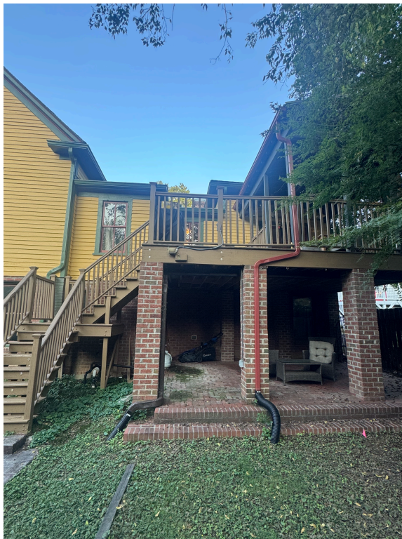
Current view of the deck and stairs. Updated footprint will remove rotted deck and bring stairs down onto the existing brick patio
