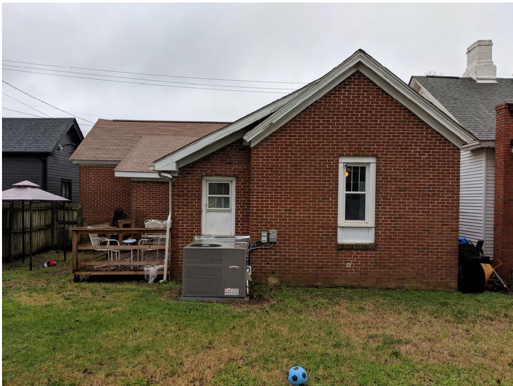
Rear Elevation Rear gable and shed roofs to be demolished.
