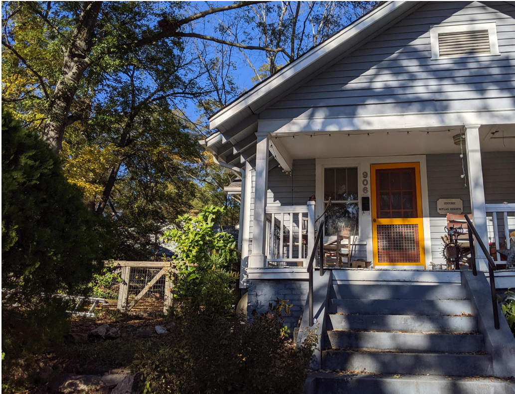
WOOD/WIRE MESH FENCE- 906 W. LENOIR STREET
