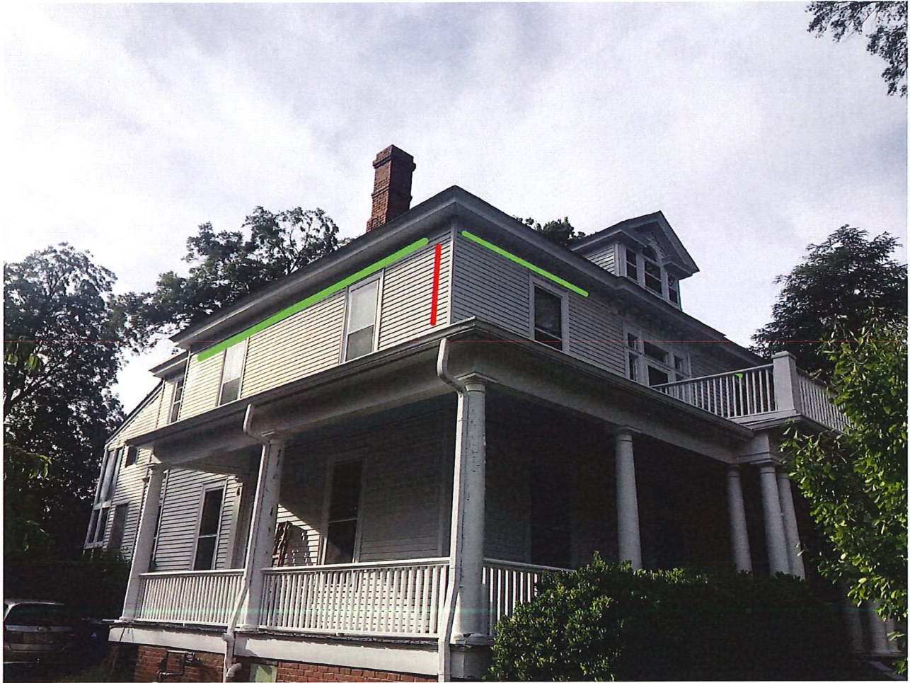
South East Corner View. Green gutters are on the top roof, red downspouts for new work and will join existing downspouts.
