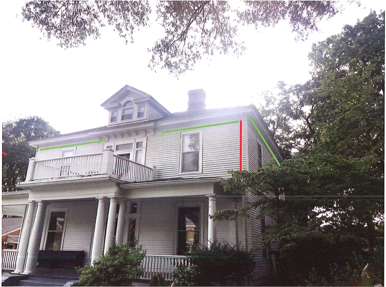
North East Corner View. Green gutters are on the top roof, red downspouts for new work and will join existing downspouts.
