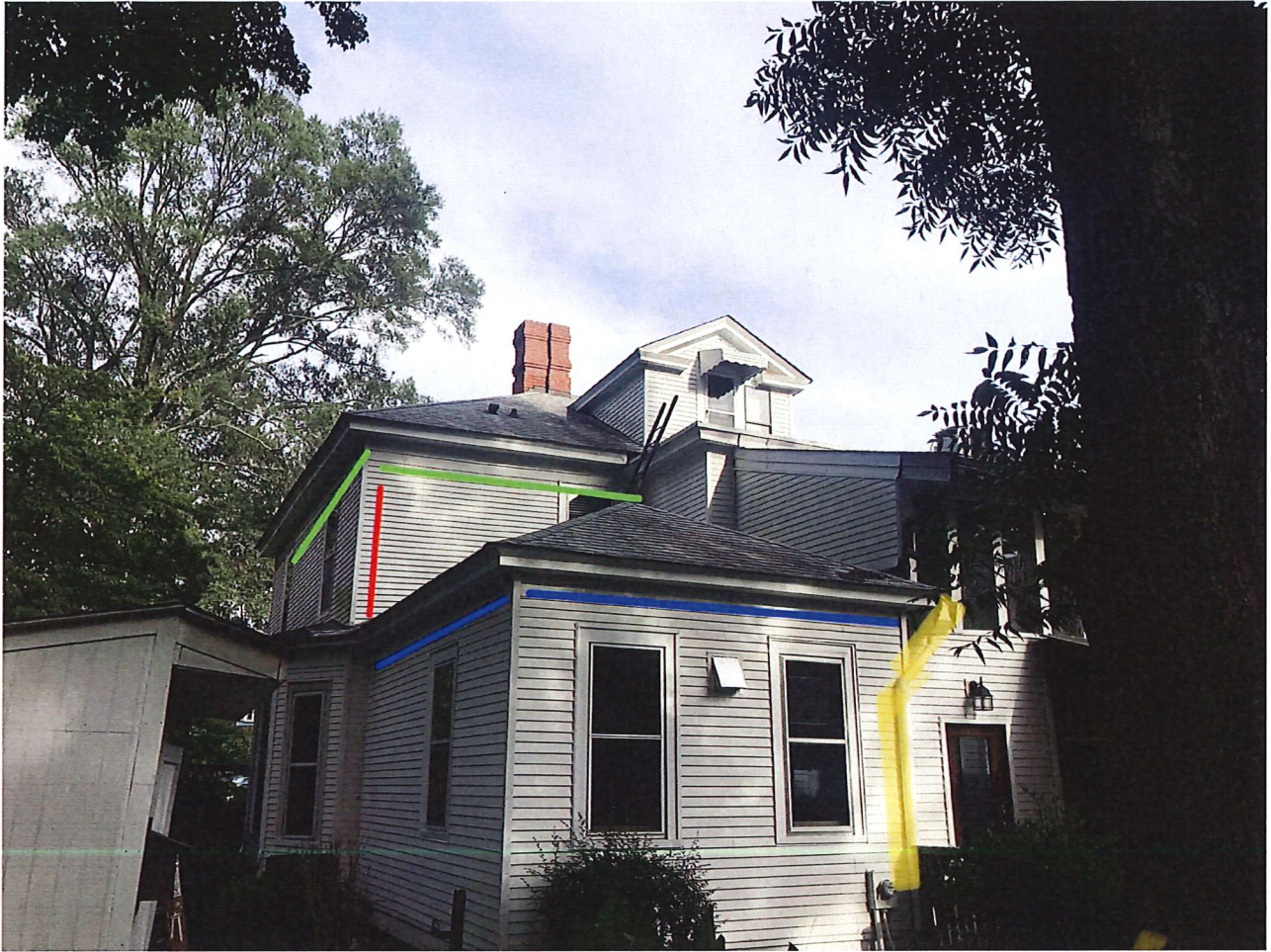
North West View. Green gutters are on the top roof, blue gutters are on the kitchen roof, red downspouts for new work, yellow downspout is existing.
