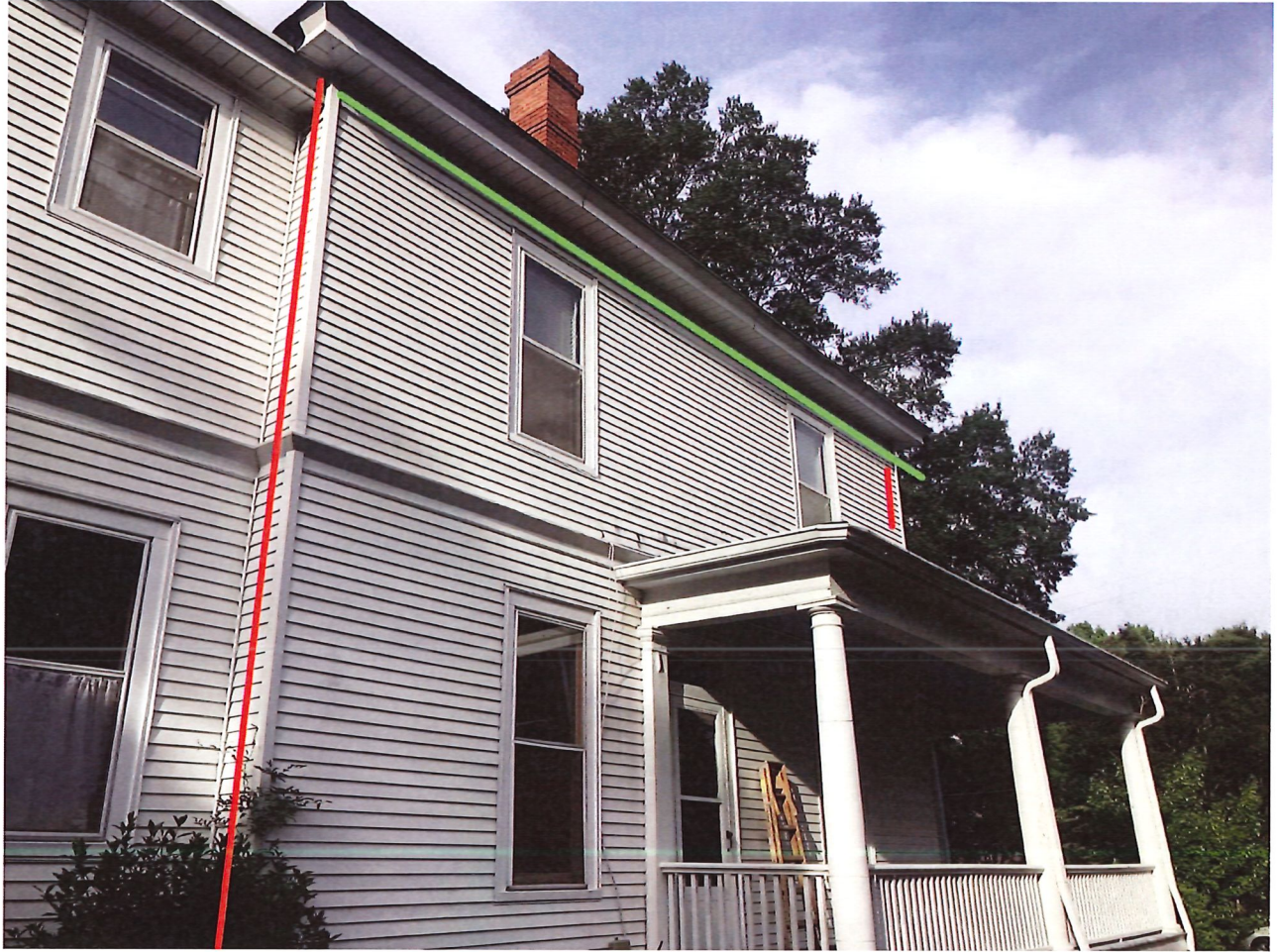
South West Corner View. Green gutters are on the top roof, red downspouts for new work and will join existing downspouts on the porch, directly to ground on the left. The rear (left) downspout will be behind the inset wall, shielded from view from the street.
