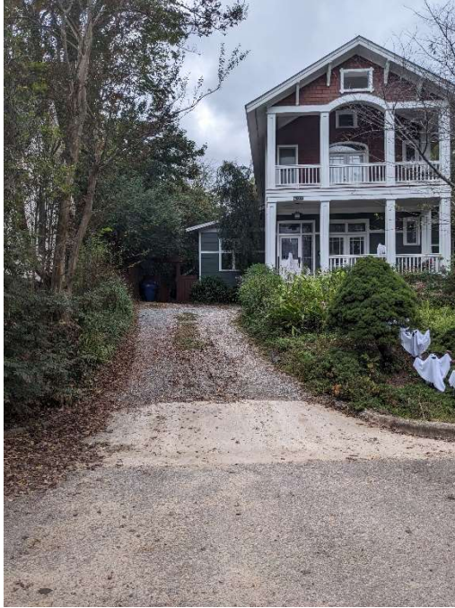
Existing damaged and overgrown driveway at 601 Leonidas Ct.
