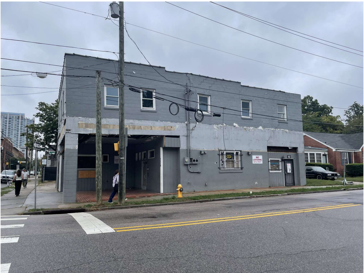
SOUTH FACADE (FACING LENOIR ST)
