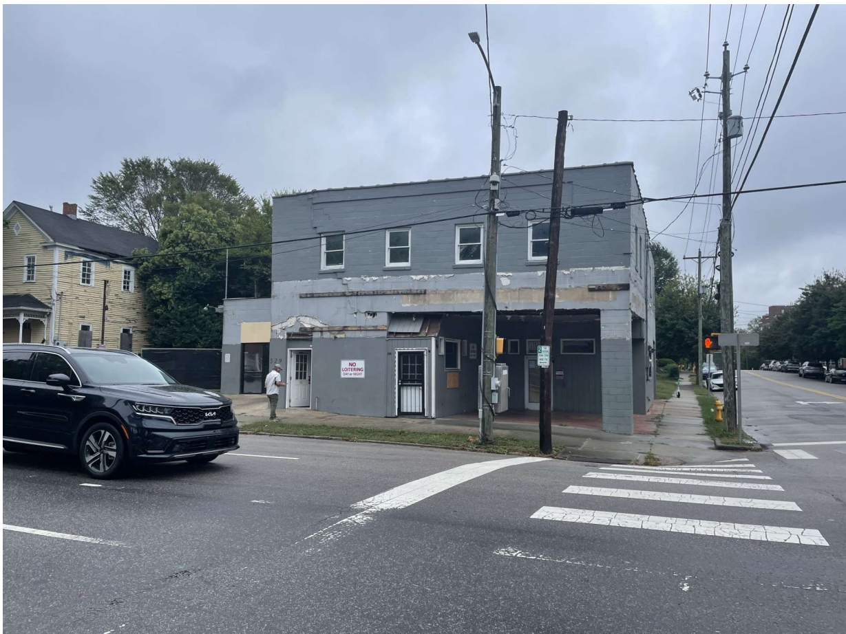
WEST FACADE (FACING BLOUNT ST)
