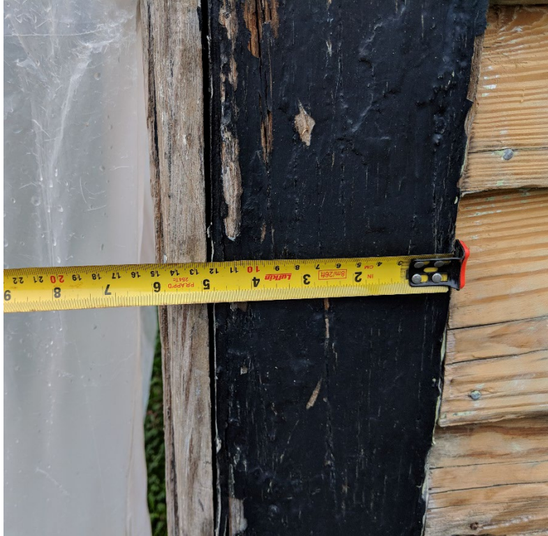
Figure 13: Corner Trim with Quarter Molding
