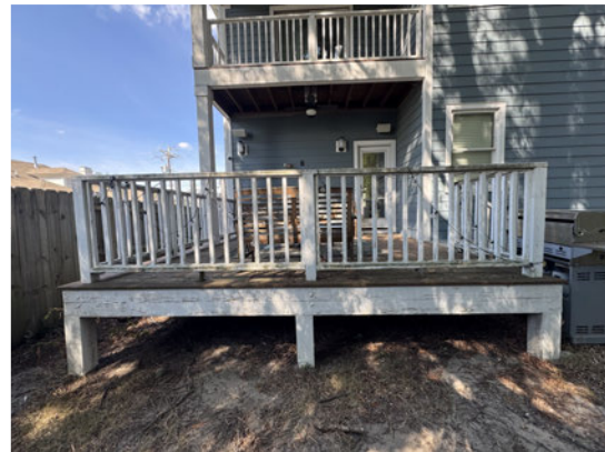
Figure 4 Existing deck IMG_7744
