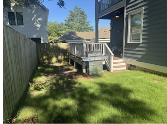
Figure 2 Existing deck, stairs and yard IMG_7403
