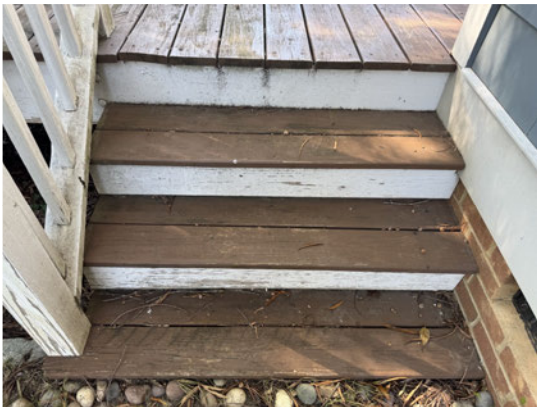
Figure 3 Existing stair treads and risers IMG_7743
