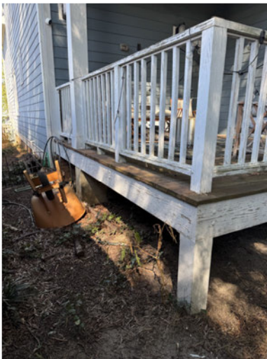
Figure 5 Existing deck IMG_7745
