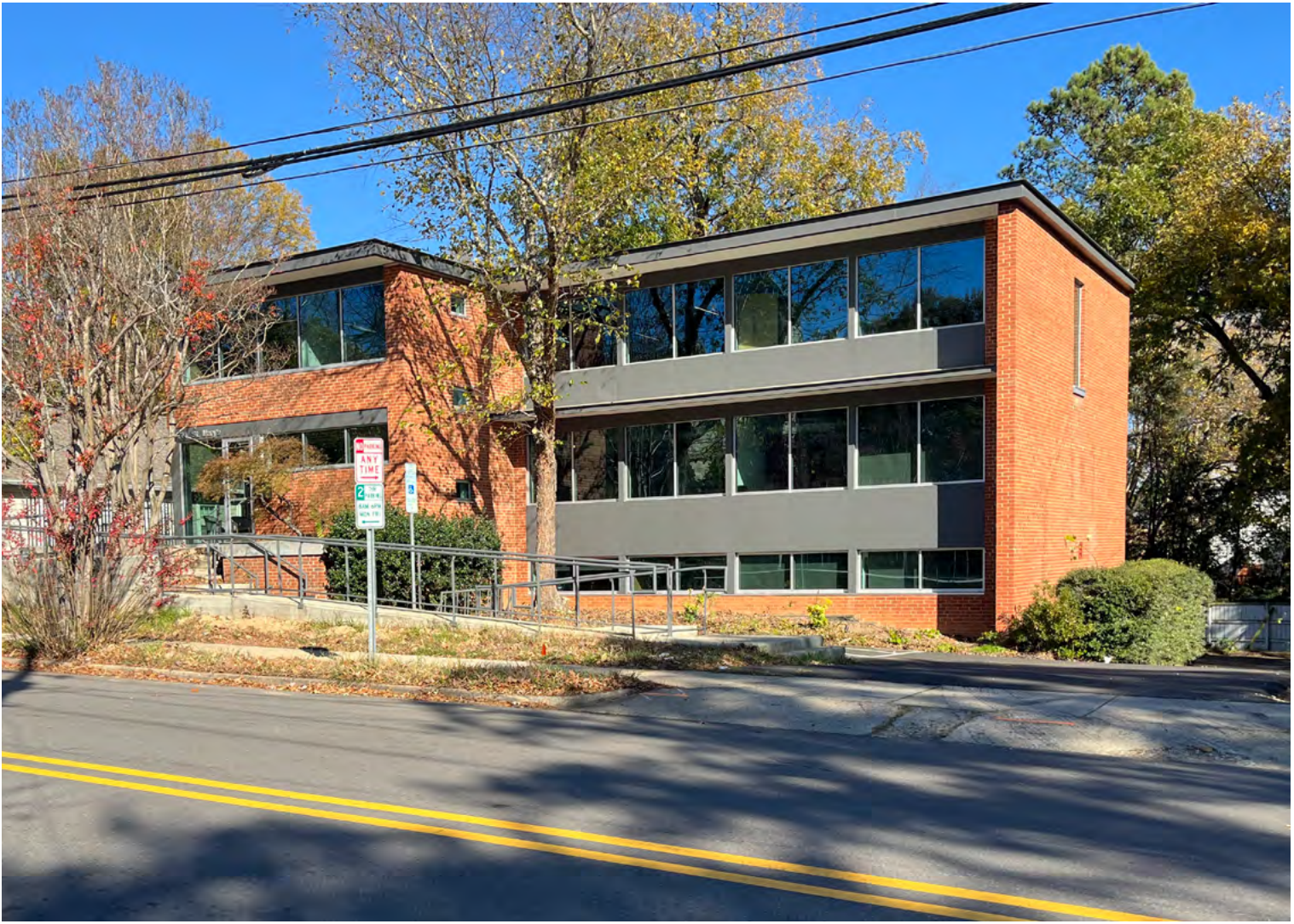
SOUTHWEST CORNER - CURRENT
