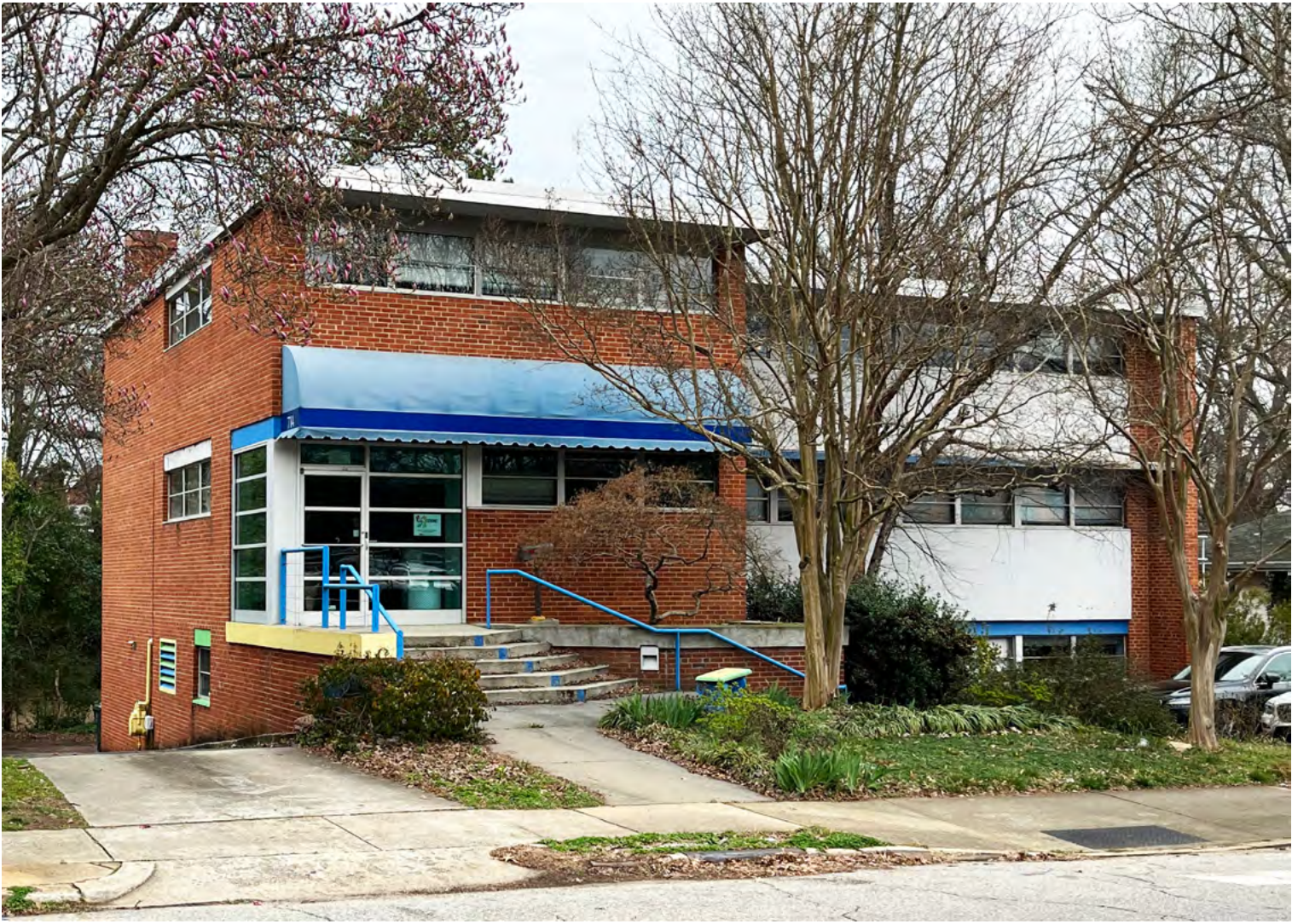
NORTHWEST CORNER - BEFORE CONSTRUCTION
