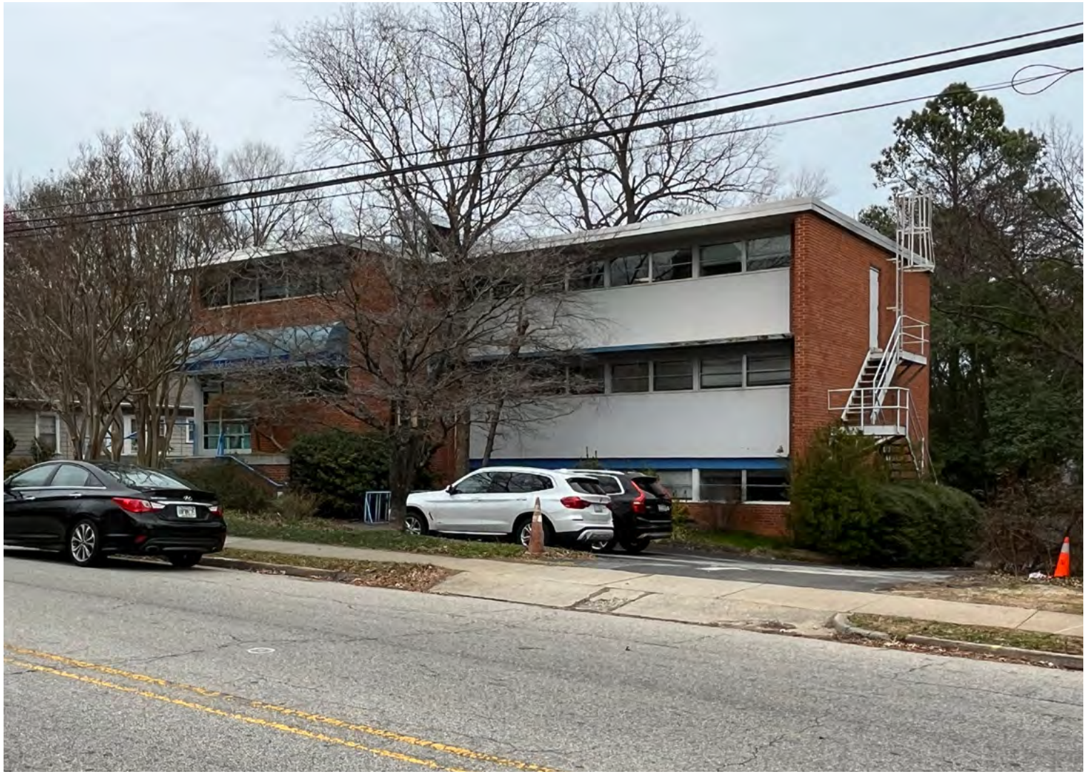
SOUTHWEST CORNER - BEFORE CONSTRUCTION
