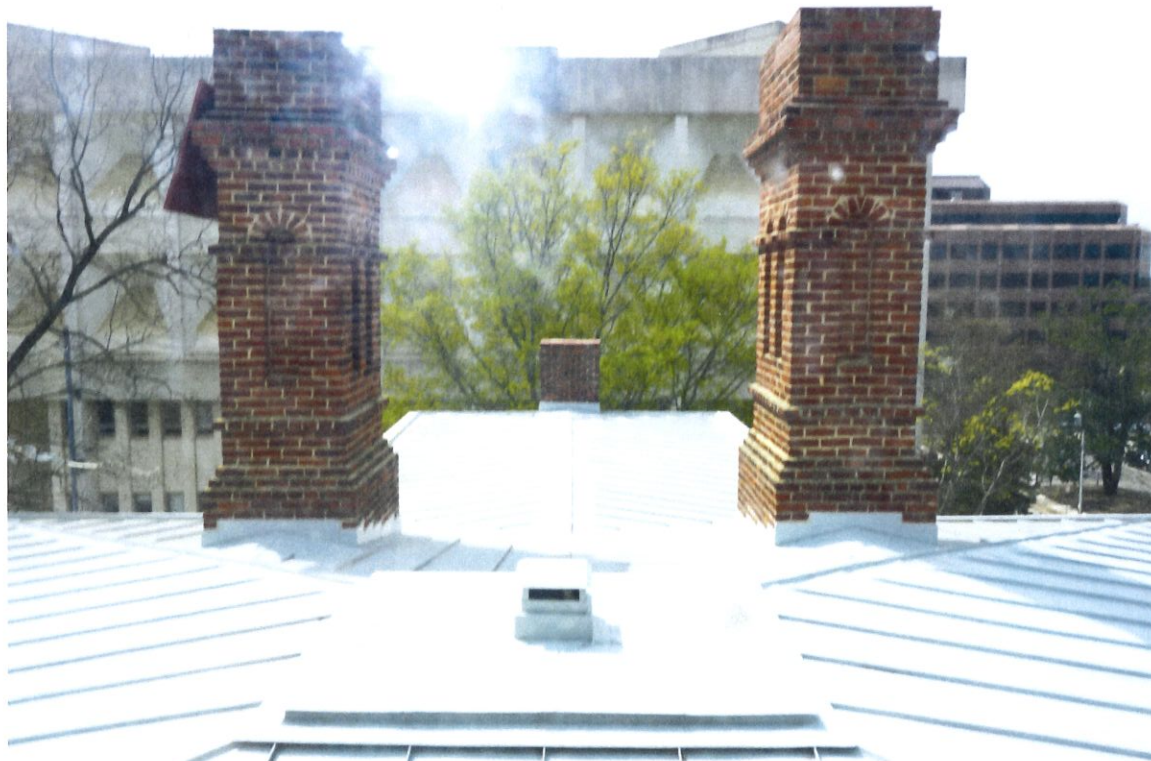
Existing Heck-Andrews House Standing Seam Roof Color And Profile
