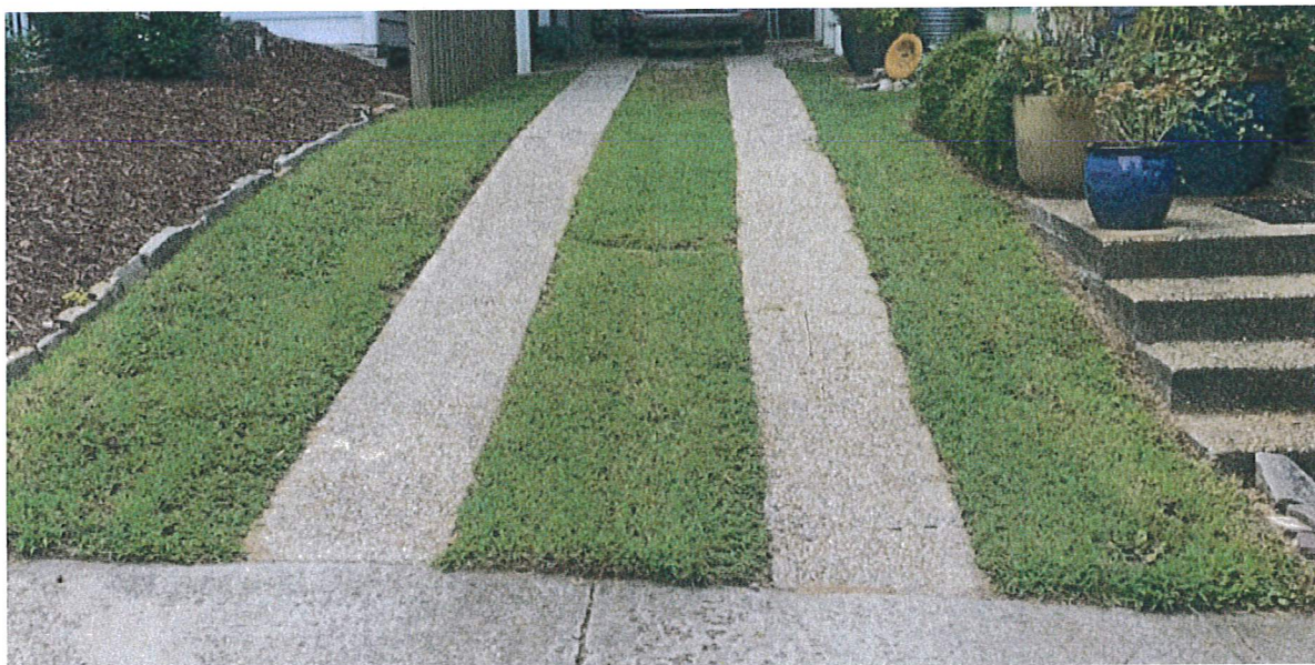
Sample washed ribbon strips separated by grass at 217 N Bloodworth St (one block north)
