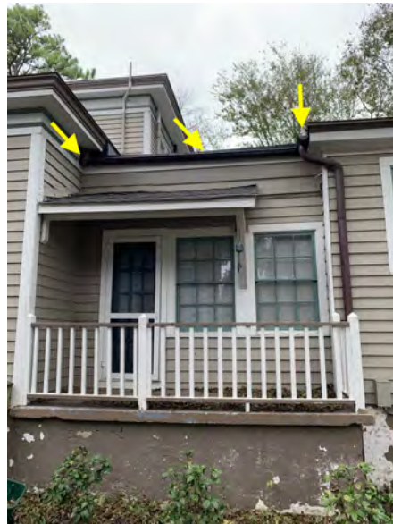
East side of connecting structure. Gutter system marked by yellow arrows.
