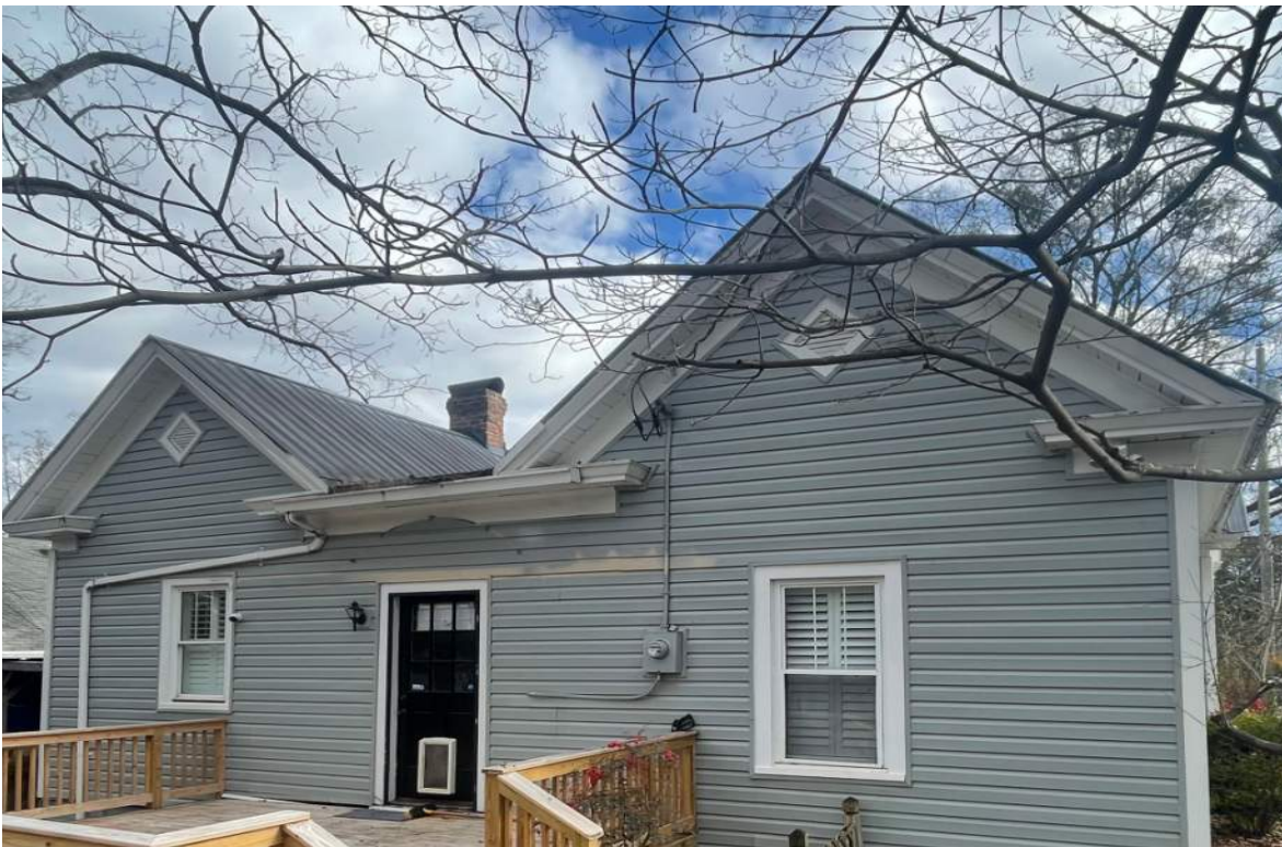
10- Existing south elevation gable details
