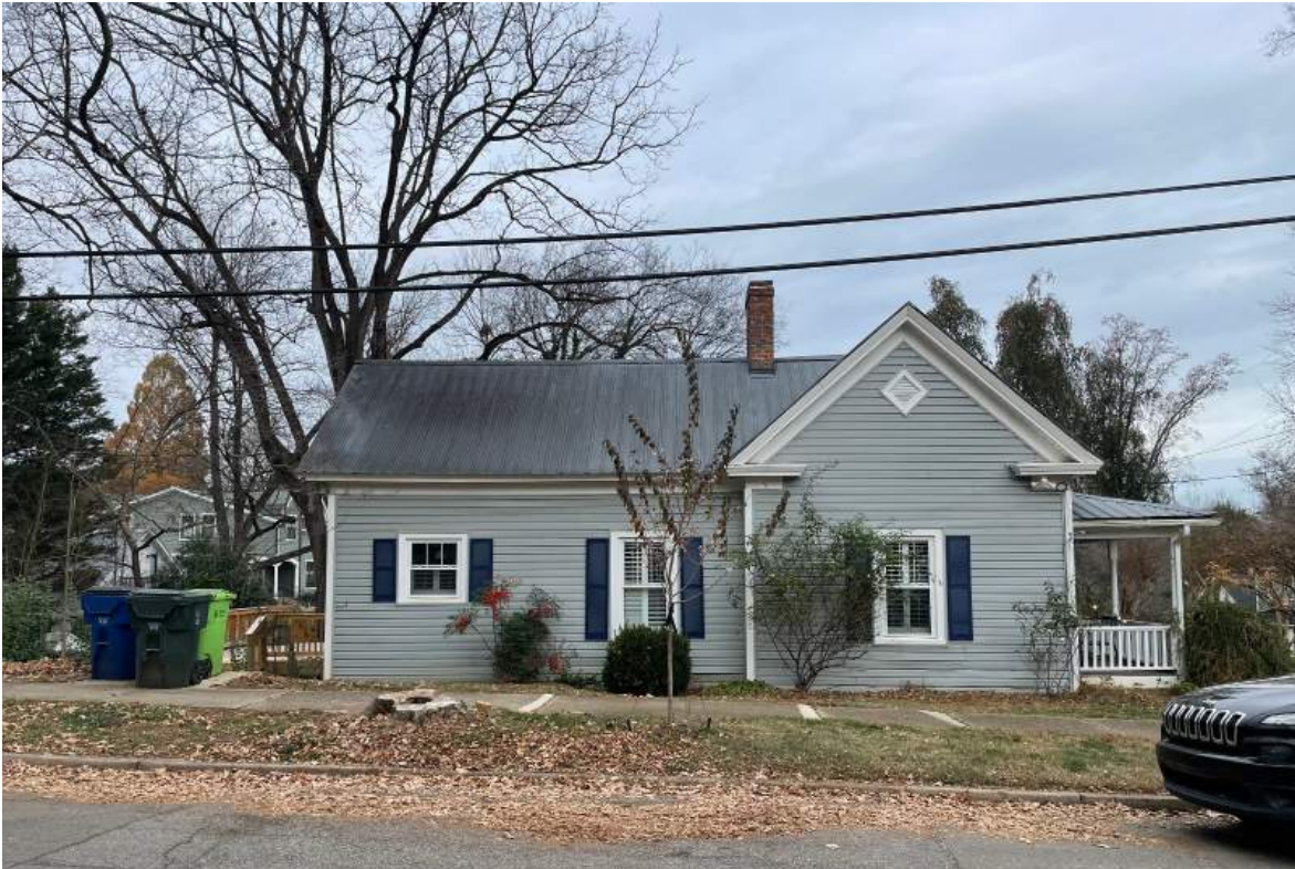
03- Existing south elevation from Jefferson Street
