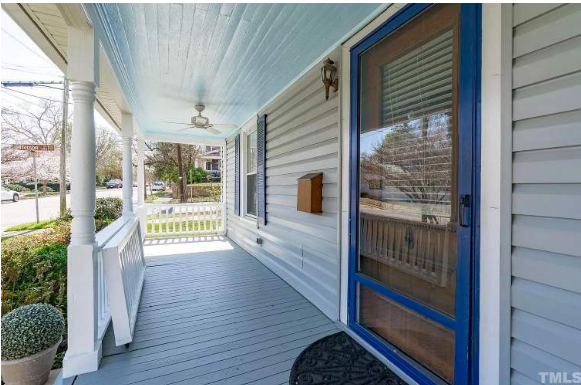
06 - Existing North view Front Porch
