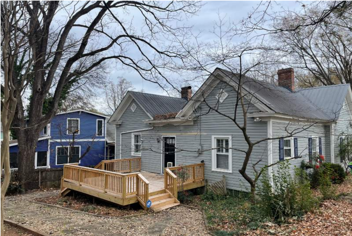
07- Existing southwest view from Jefferson Street/ Rear Elevation
