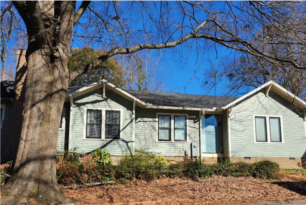
01- 1100 Filmore Street- Connected new addition with glassed in portion, gabled addition-dropped 1' below original
