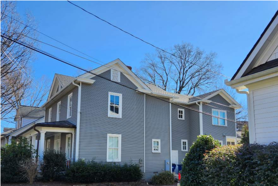
03- 507 Devereux Street- Connected new addition with connector below original eave height, recessed from existing structure
