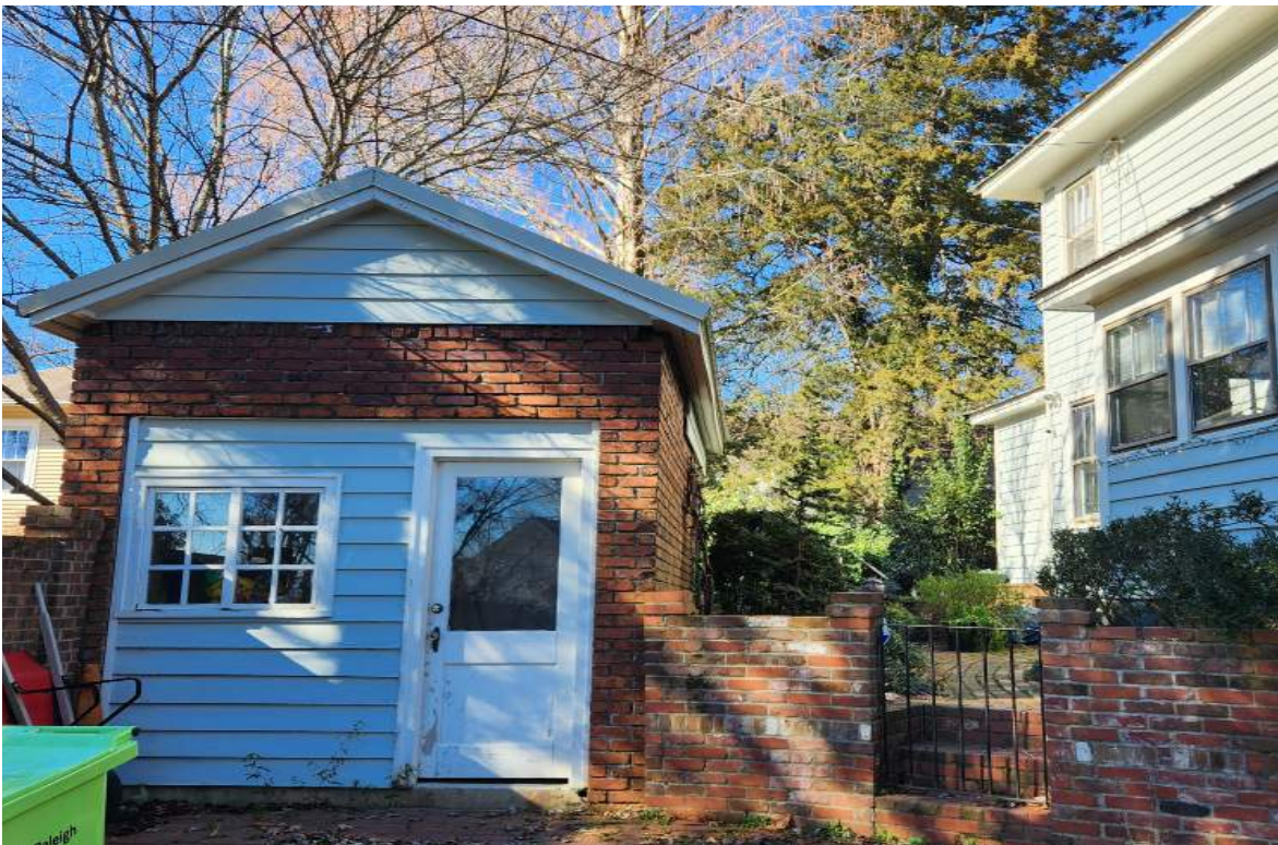
04- 517 Cole Street Original outbuilding use of brick as exterior wall despite original house being lap siding.
