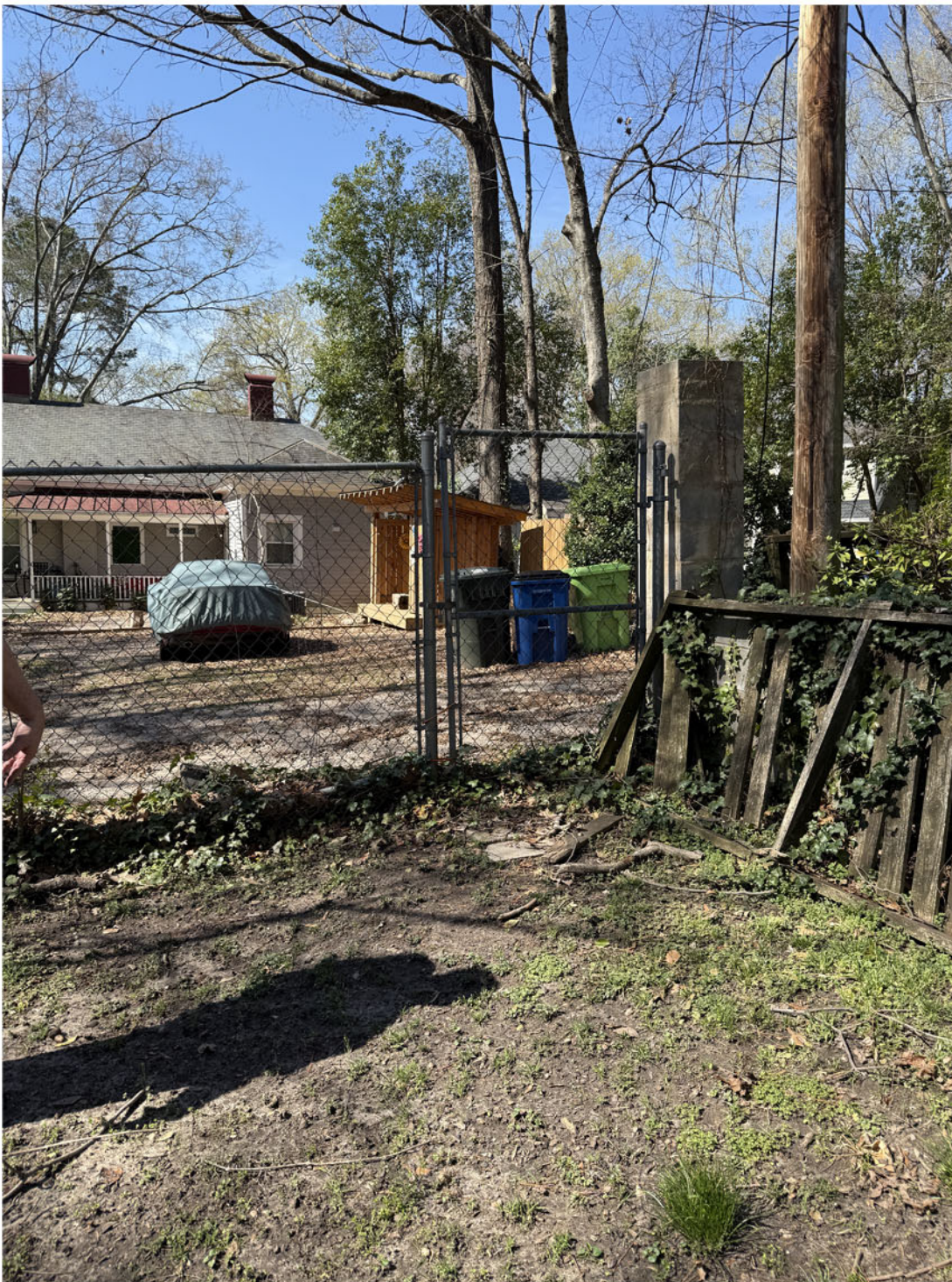
Back corner of the lot where a brick dry laid pad will be installed for trash cans and access to existing gate
