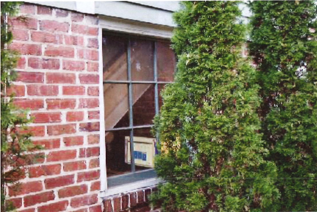
Inset, non-operable basement window to receive picture window.
