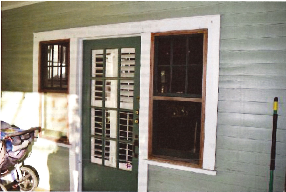
Two windows flanking front door will receive operable storm windows.
