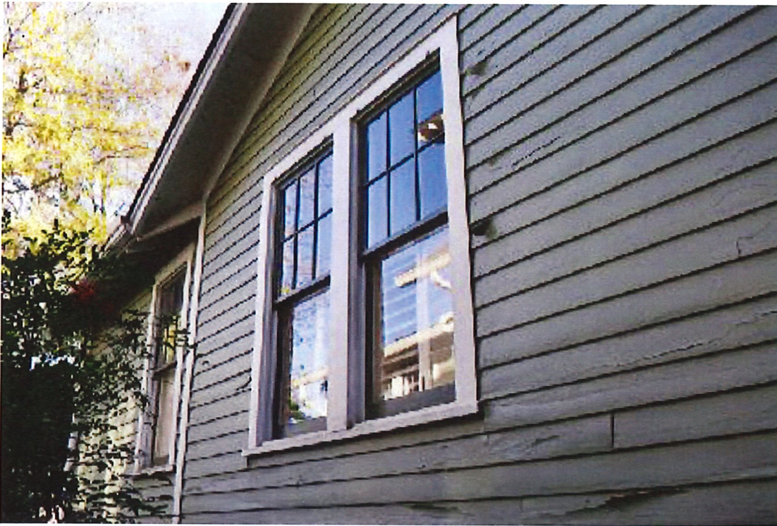
Windows in dining room to receive operable storm windows. Left-most window in coat closet to receive picture window.
