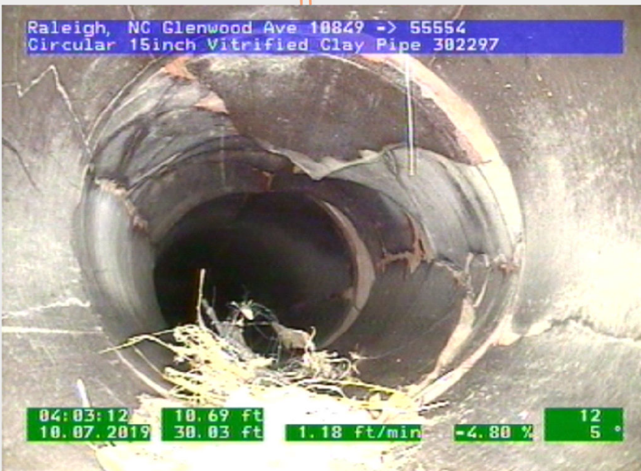
Vitrified Clay Pipe - Poor Condition
