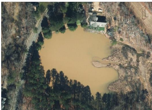
Aerial view of Camp Pond Dam and Richland Drive
