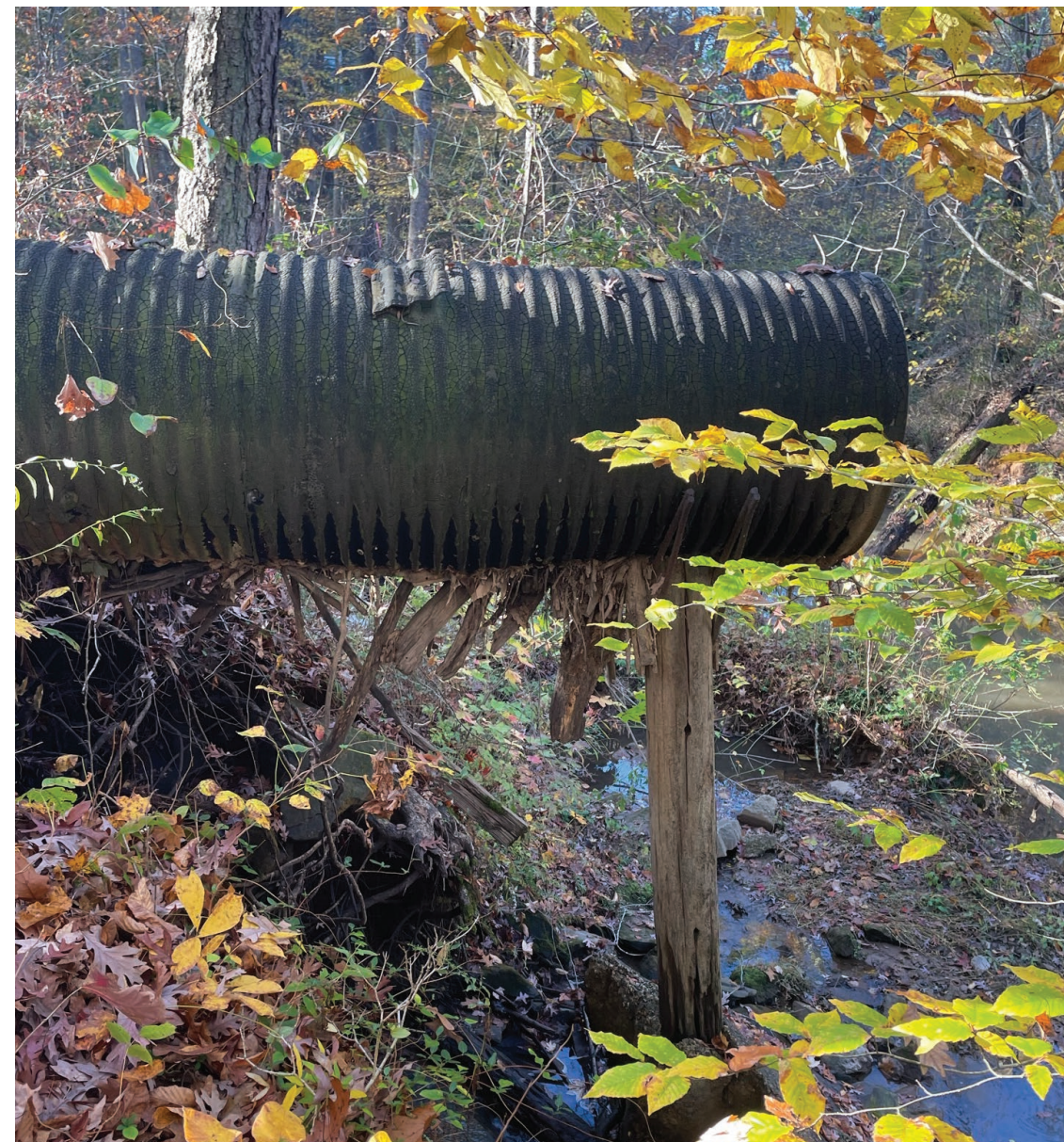
Figures 4 and 5: Principal spillway pipe is deteriorated due to rust.
