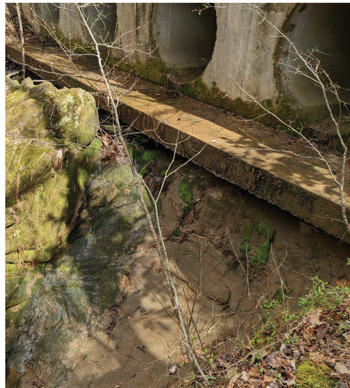
Figure 2: Loss of bedding material.
