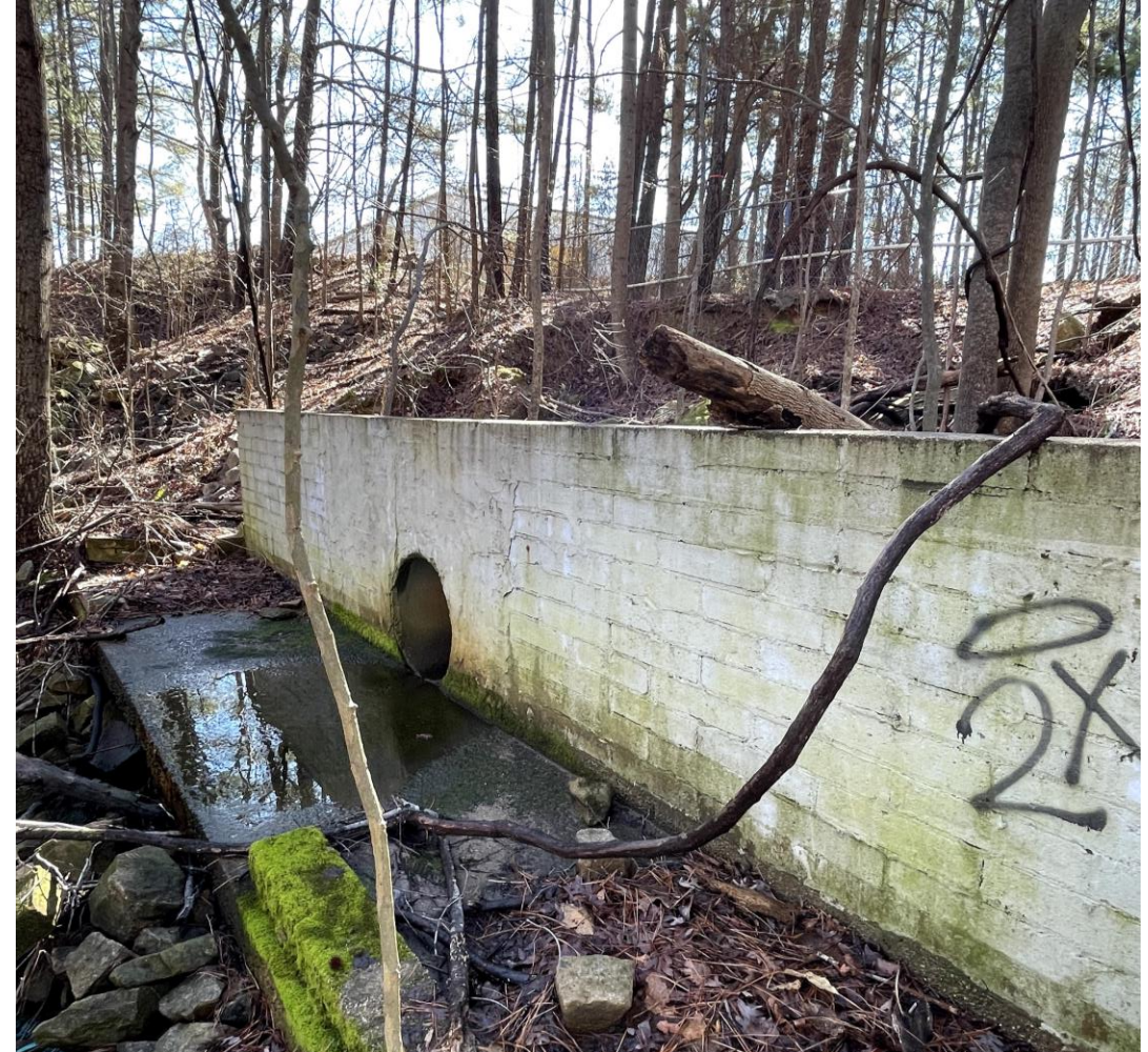
Figure 2: Pipe outlet from Spottswood Street detention pond
