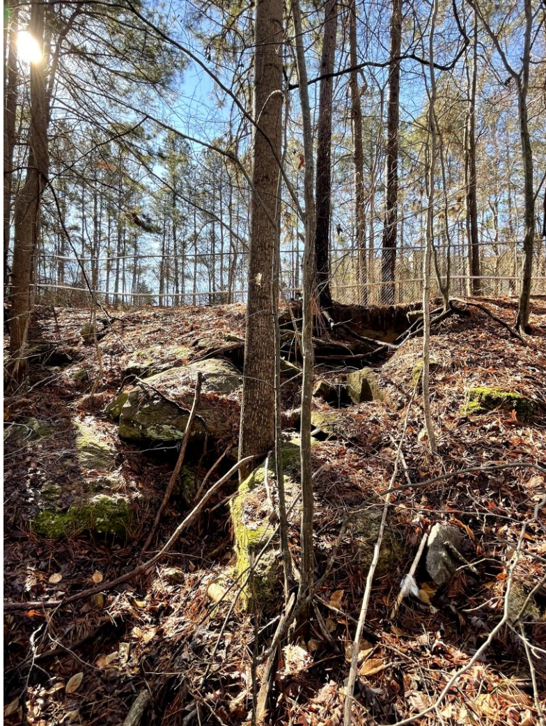
Figure 1: Steep and highly eroded slopes.
