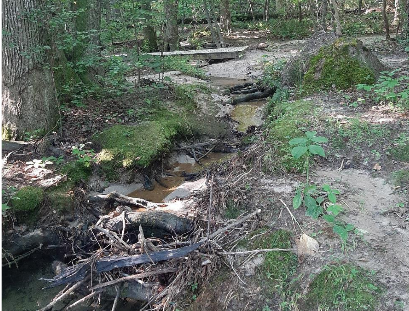
Figure 3: Banks have become incised due to high energy water flow.
