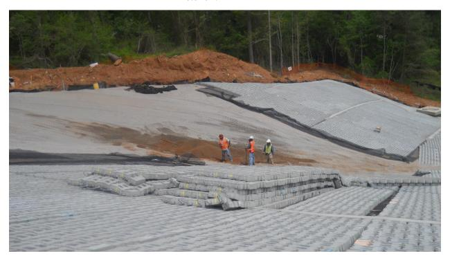
Picture 18: Installation of Overtopping Protection at Lake Johnson Dam
